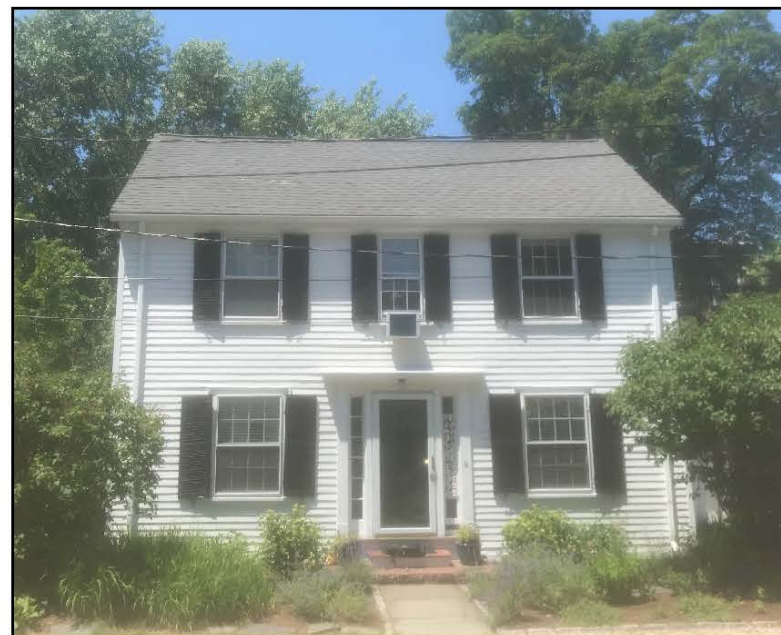
65 FOSTER ST. – RIGHT SIDE/ ENTRY ELEVATION
