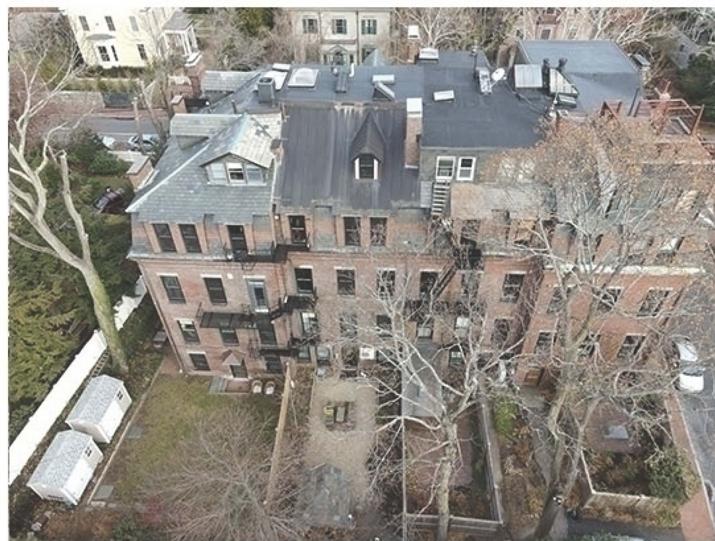
2 - REAR YARD WEST VIEW, EXISTING
