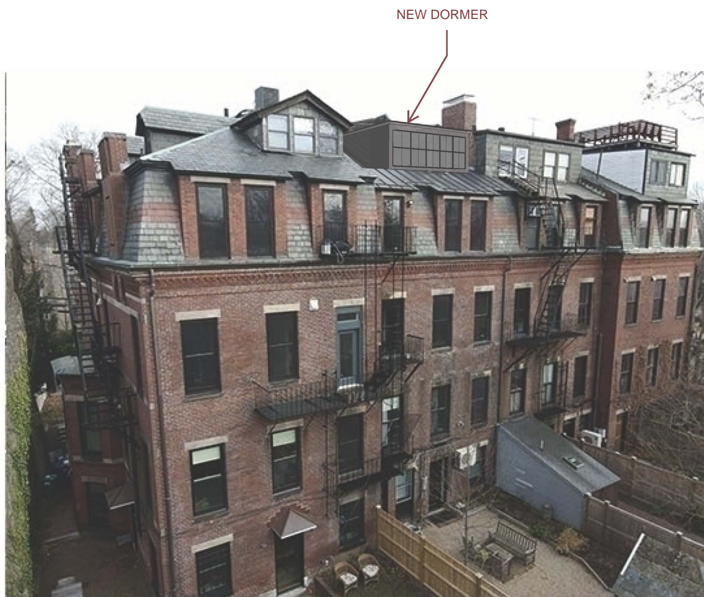
4 - NORTHWEST CORNER WITH DORMER / TERRACE
