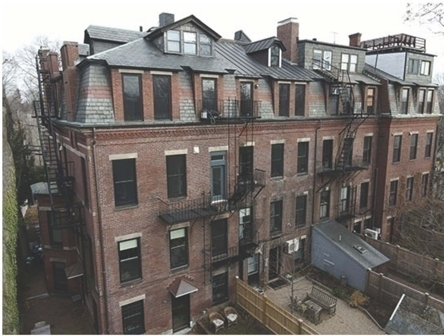
1 - NORTHWEST CORNER, EXISTING
