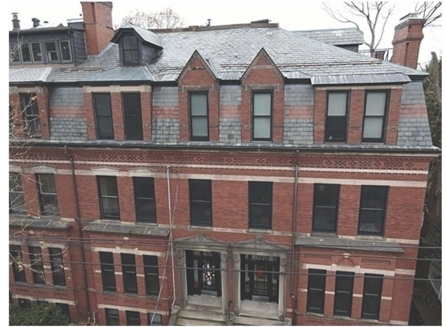
3 - VIEW UP TO ROOF, EXISTING
