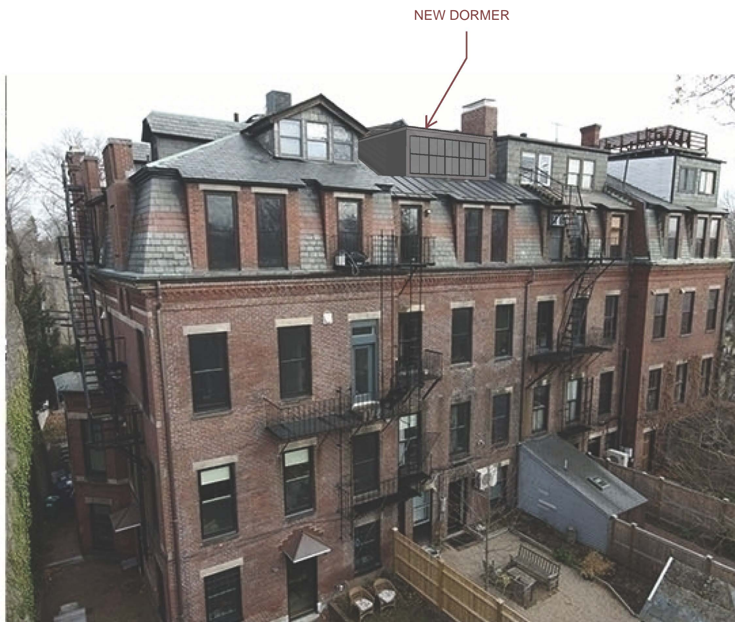
4 - NORTHWEST CORNER WITH DORMER / TERRACE
