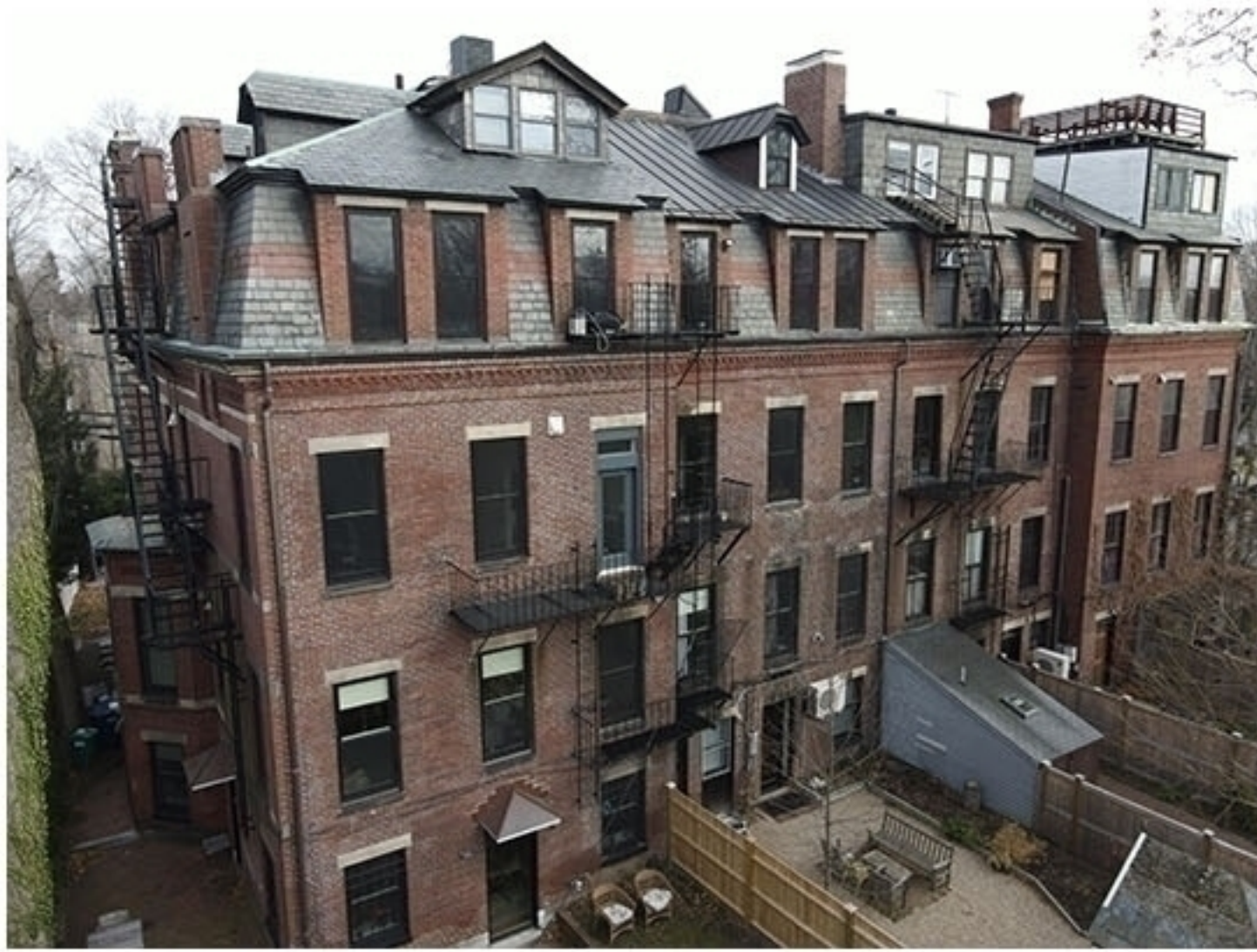
1 - NORTHWEST CORNER, EXISTING
