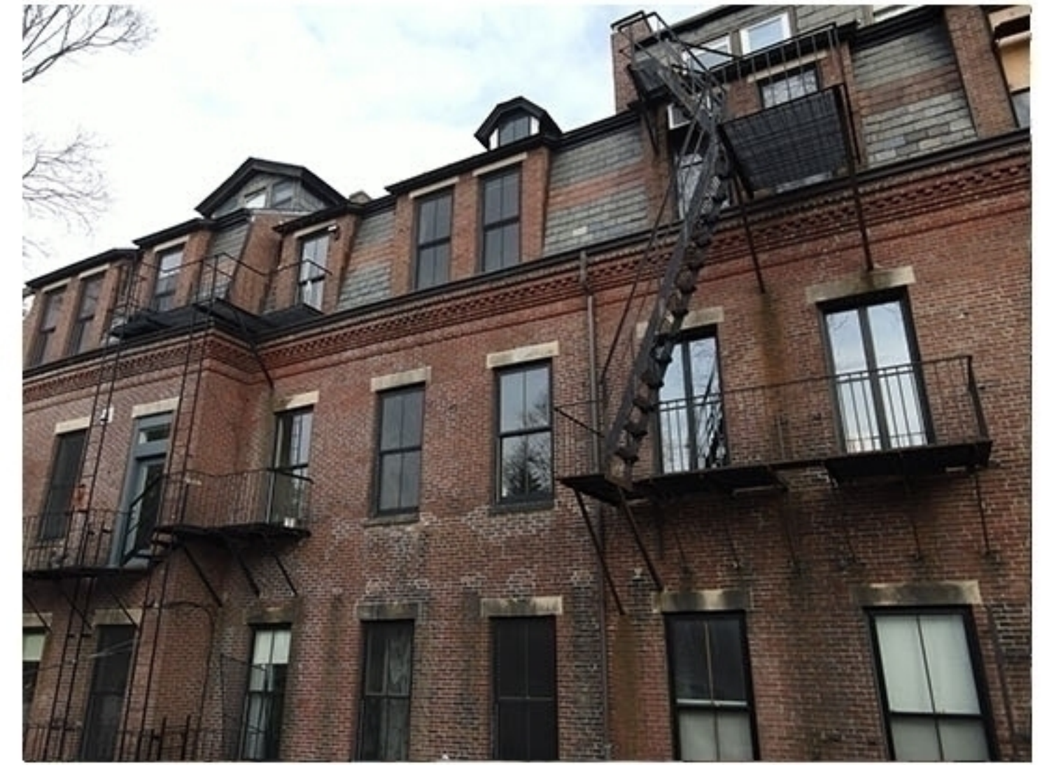
3 - REAR YARD VIEW UP, EXISTING
