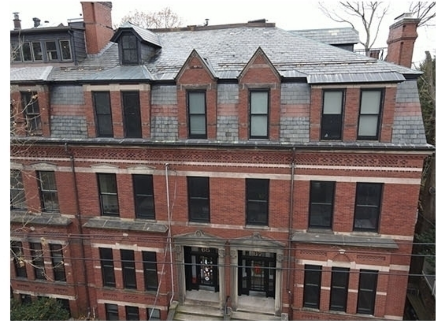
3 - VIEW UP TO ROOF, EXISTING
