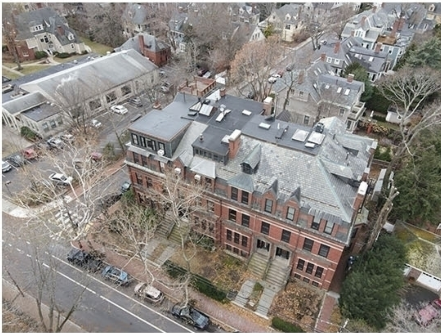
1 - VIEW FROM NORTHEAST CORNER, EXISTING
