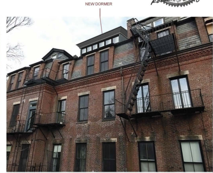
6 - REAR YARD VIEW UP WITH DORMER / TERRACE
