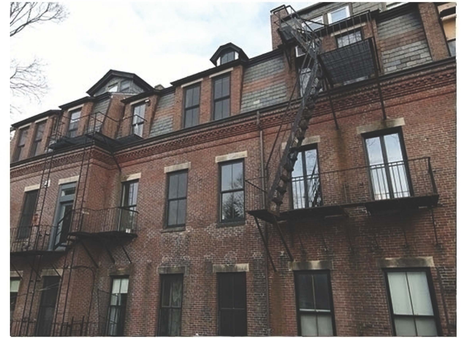
3 - REAR YARD VIEW UP, EXISTING
