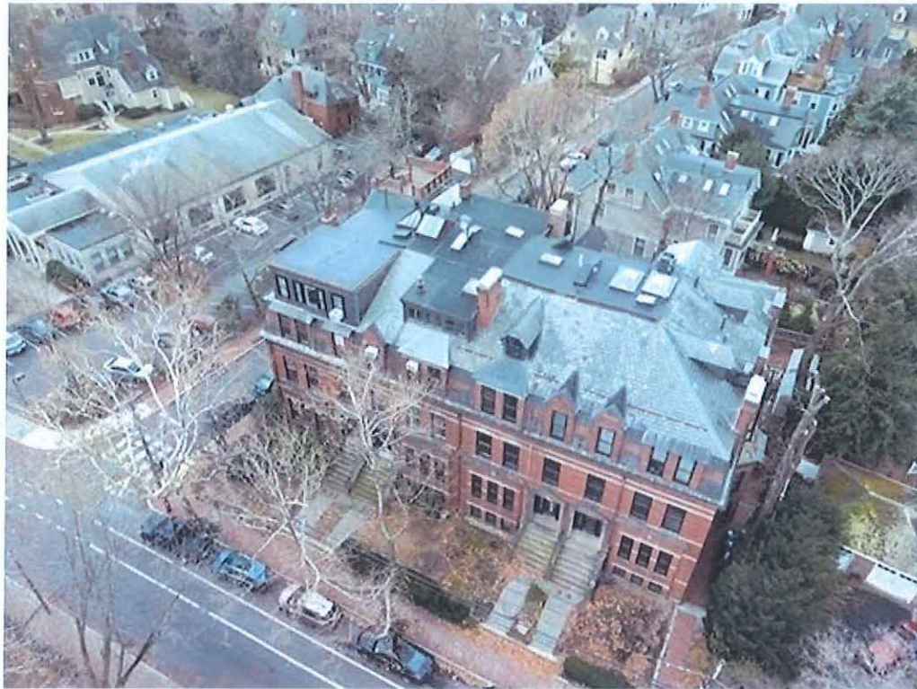
1 - VIEW FROM NORTHEAST CORNER, EXISTING
