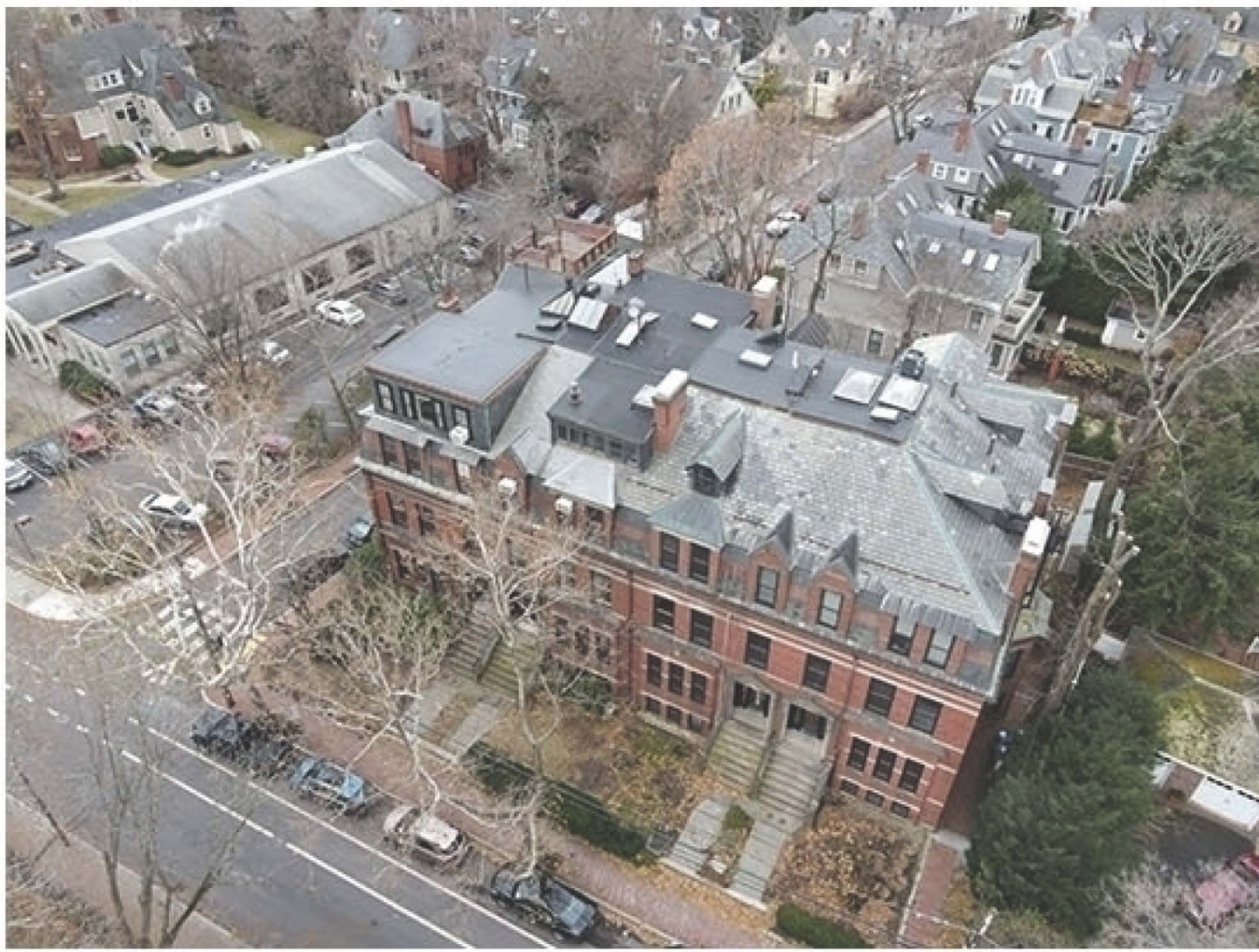
1 - VIEW FROM NORTHEAST CORNER, EXISTING
