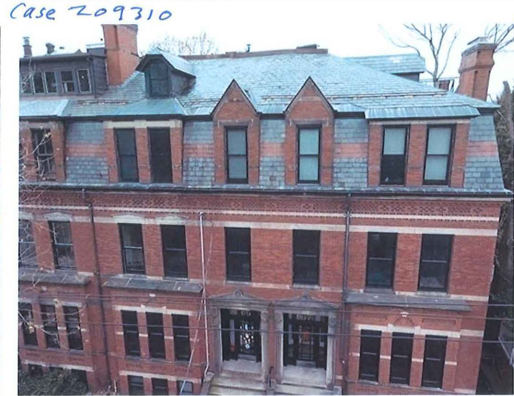
3 - VIEW UP TO ROOF, EXISTING
