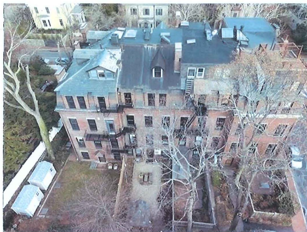
2 - REAR YARD WEST VIEW, EXISTING
