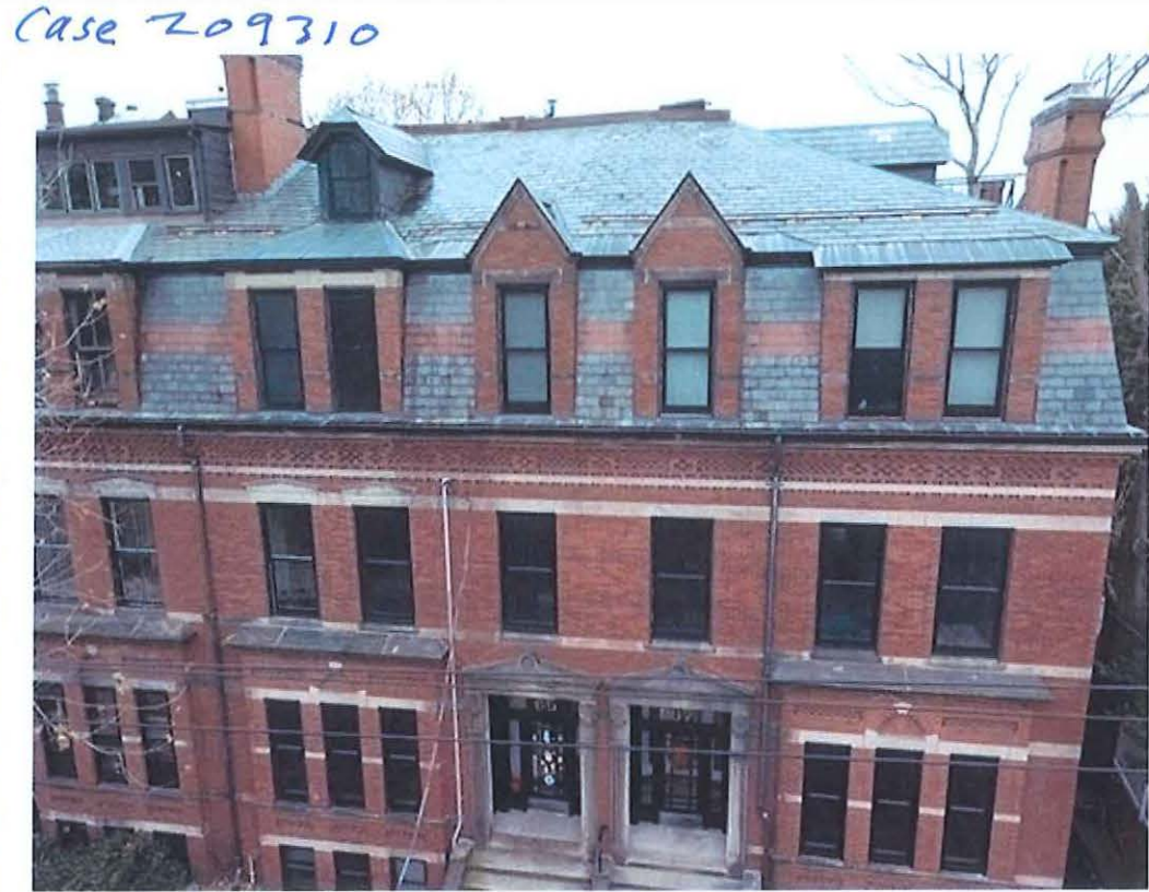
3 - VIEW UP TO ROOF, EXISTING
