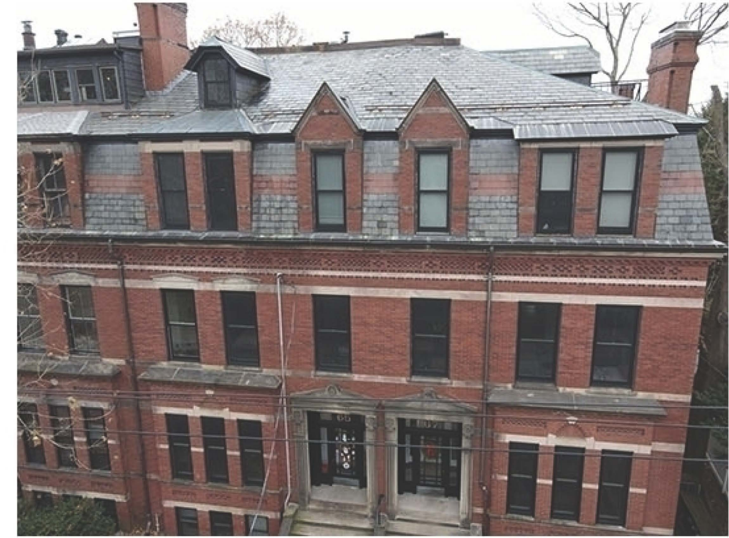
3 - VIEW UP TO ROOF, EXISTING
