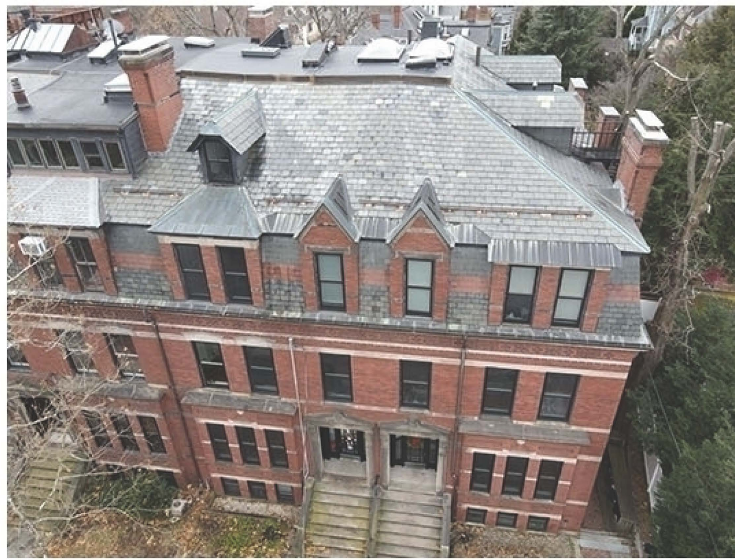
2 - VIEW FROM FRONT YARD, EXISTING
