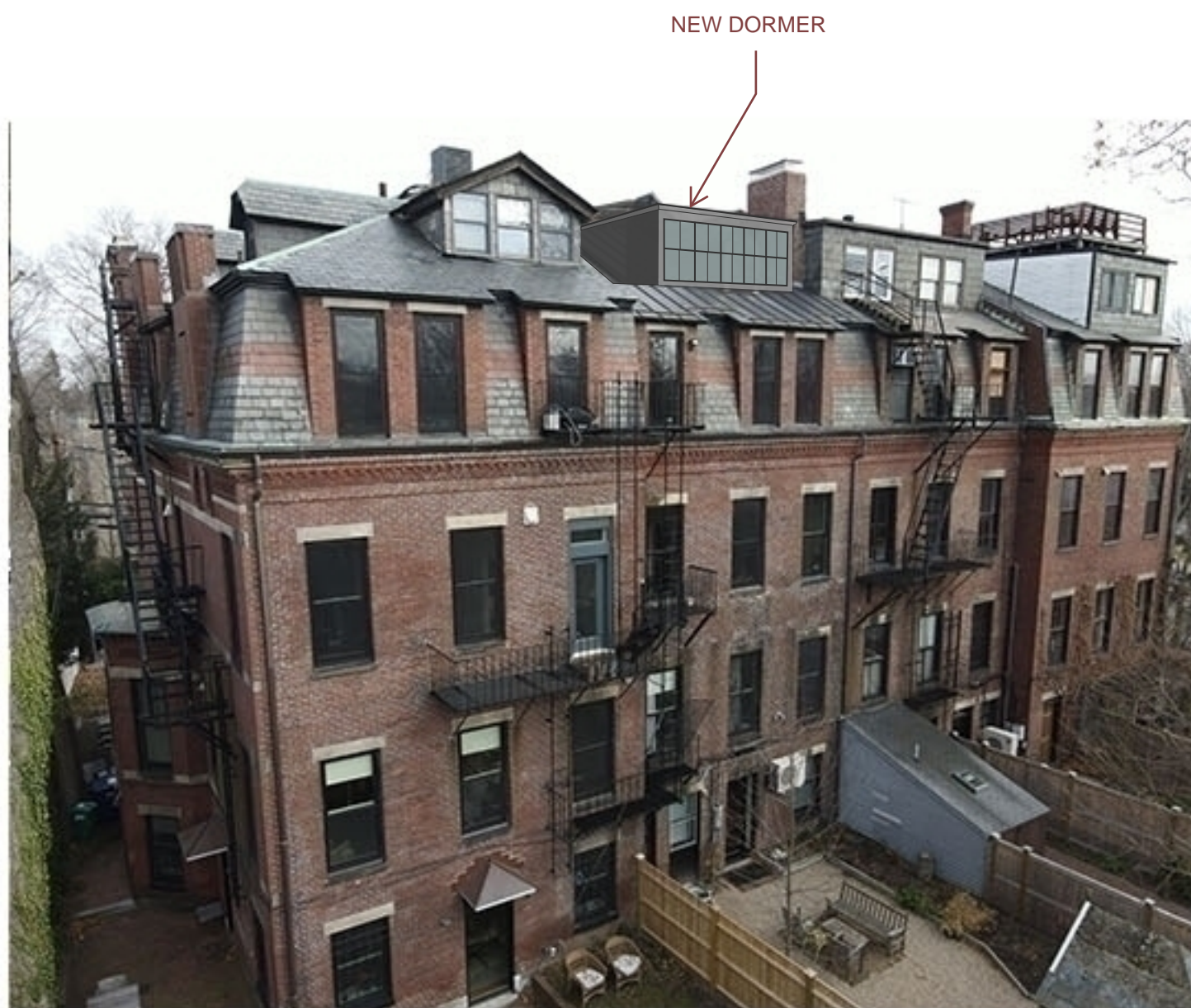
4 - NORTHWEST CORNER WITH DORMER / TERRACE
