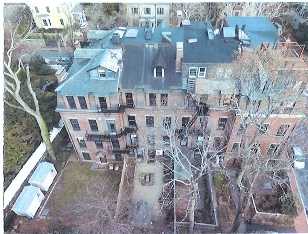
2 - REAR YARD WEST VIEW, EXISTING
