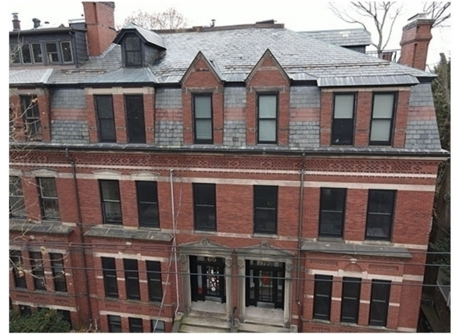
3 - VIEW UP TO ROOF, EXISTING
