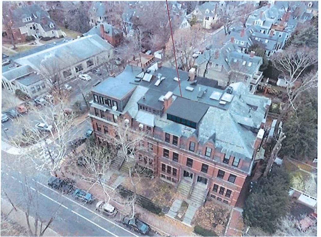
4 - VIEW FROM NORTHEAST CORNER WITH DORMER
