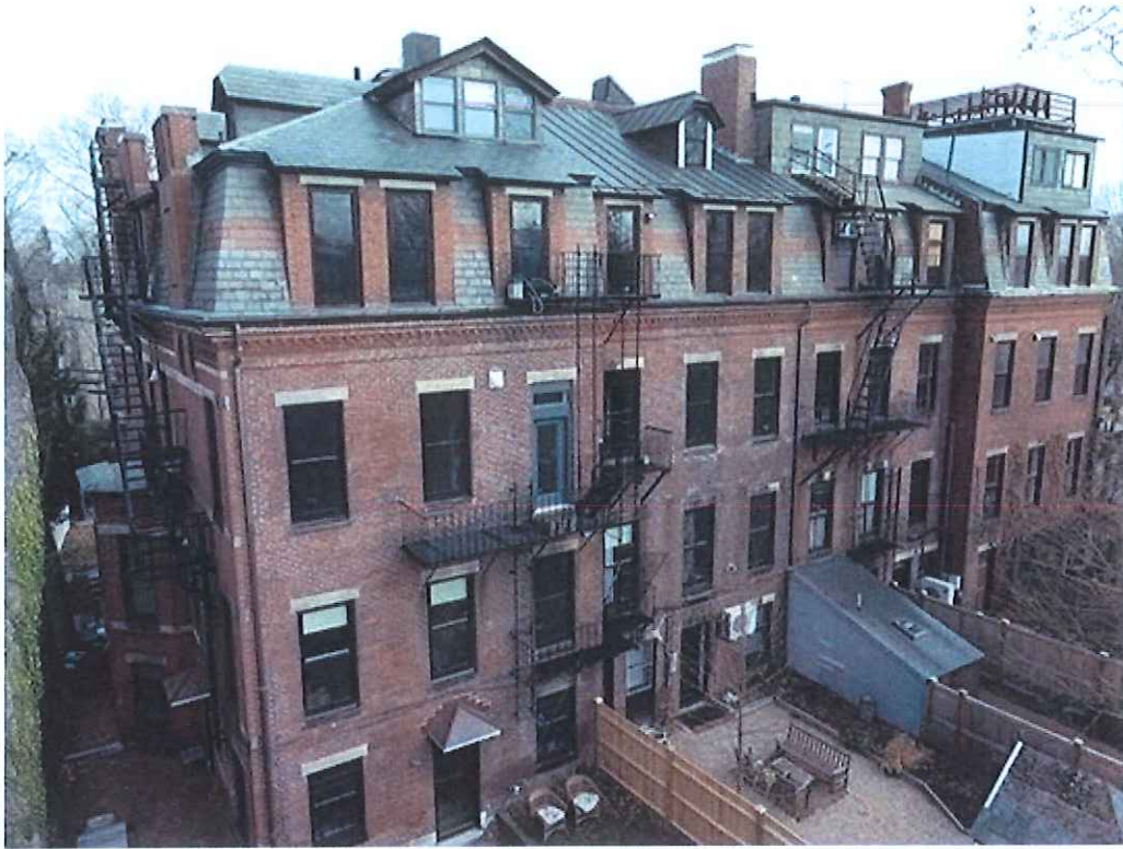
1 - NORTHWEST CORNER, EXISTING
