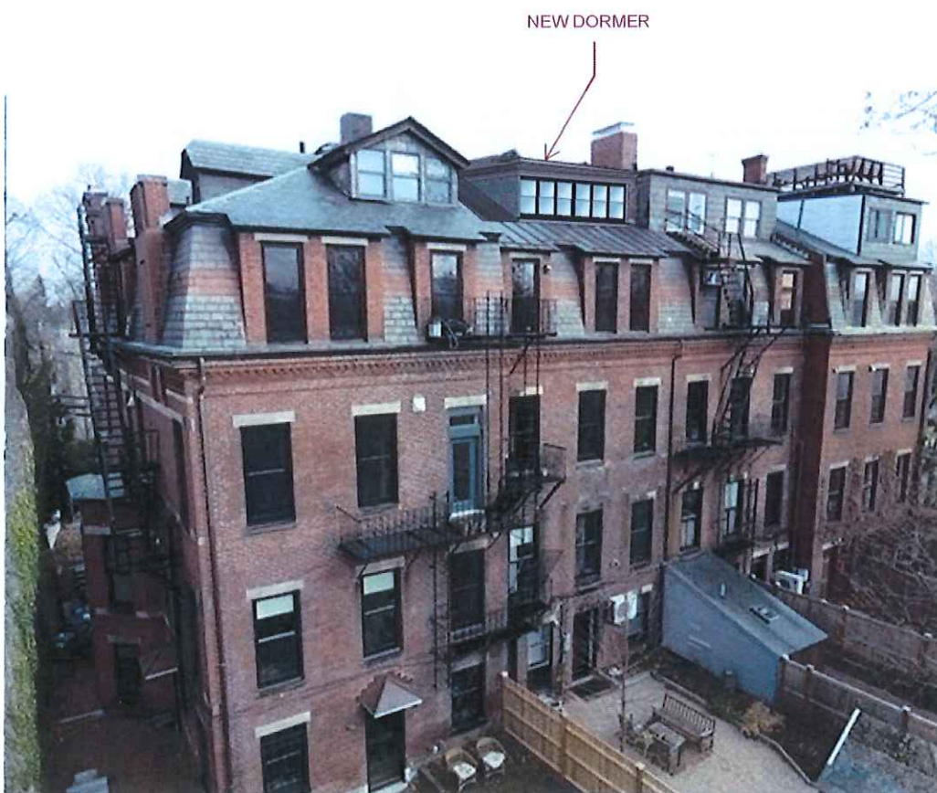
4 - NORTHWEST CORNER WITH DORMER / TERRACE
