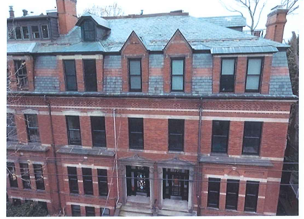
3 - VIEW UP TO ROOF, EXISTING
