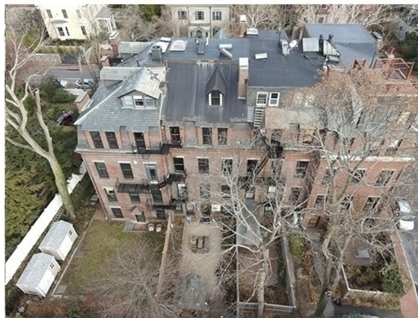
2 - REAR YARD WEST VIEW, EXISTING
