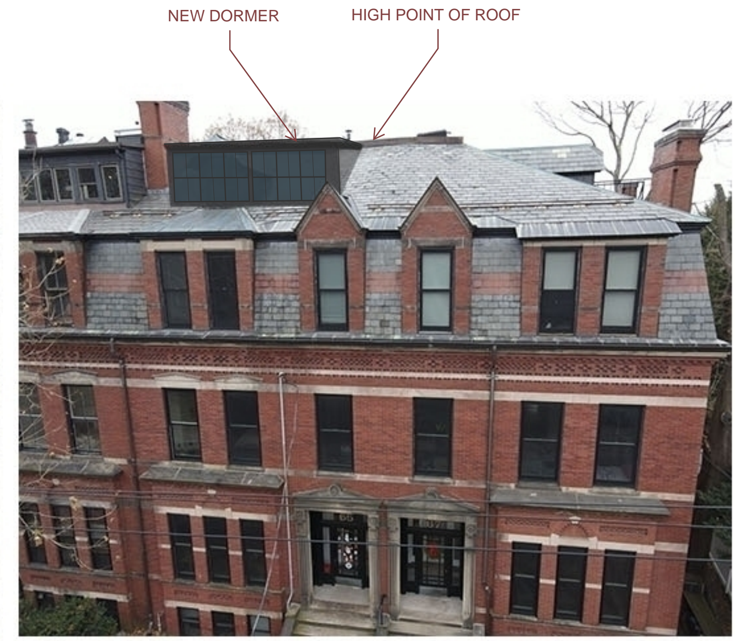
6 - VIEW UP TO ROOF WITH DORMER
