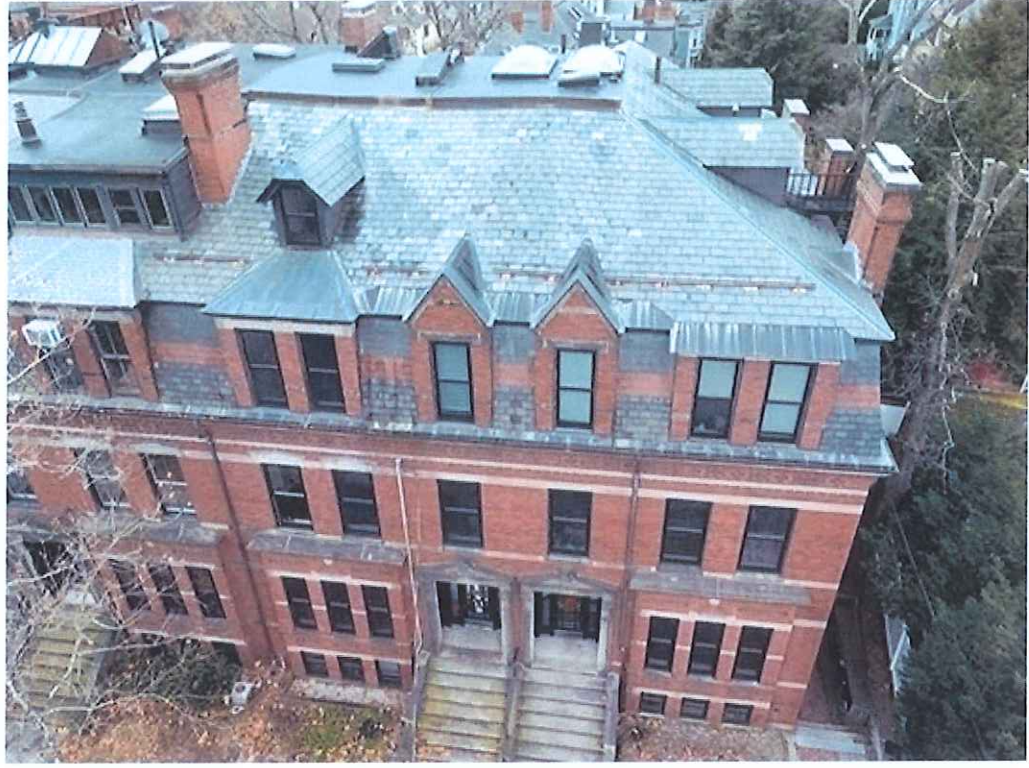
2 - VIEW FROM FRONT YARD, EXISTING
