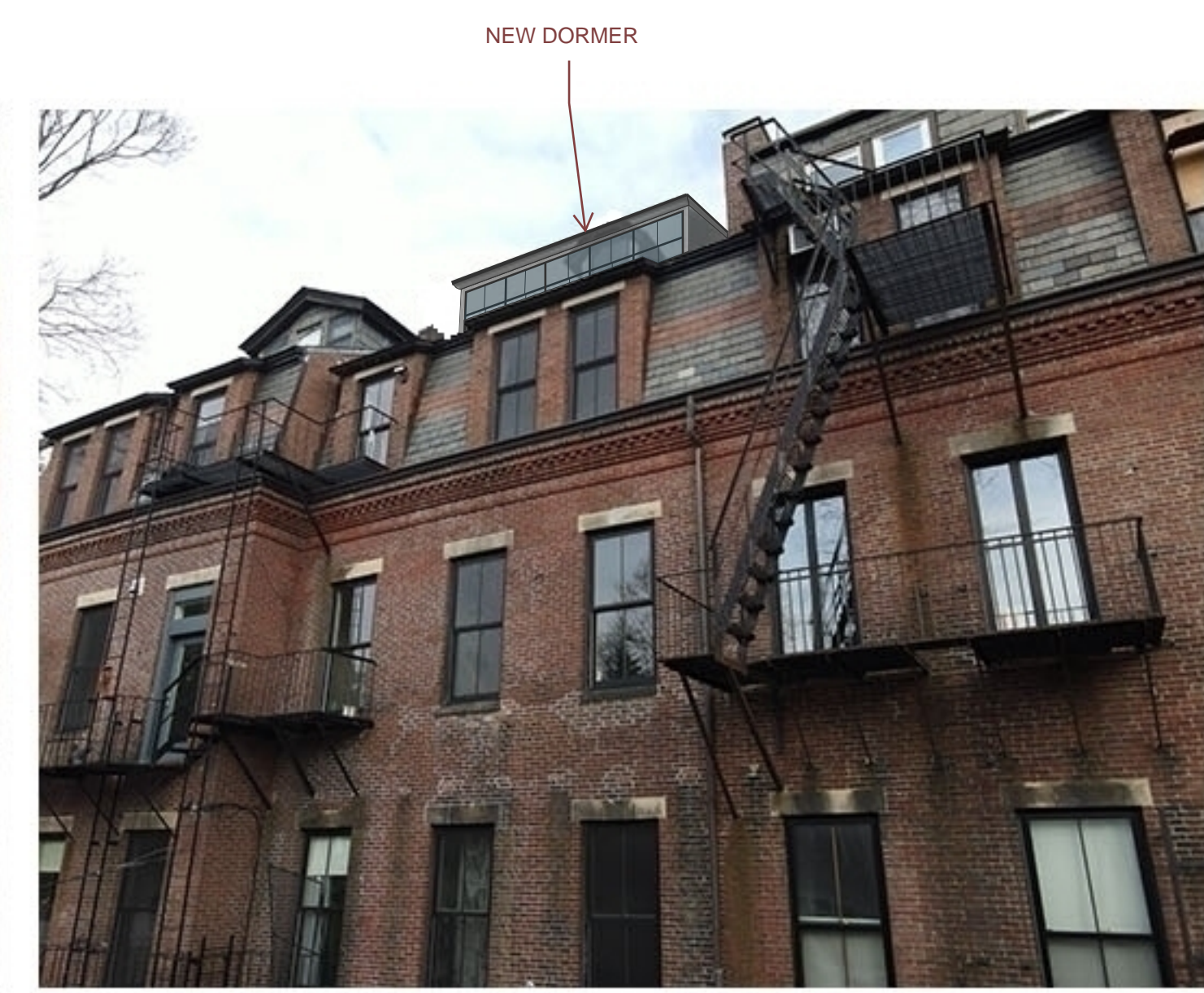
6 - REAR YARD VIEW UP WITH DORMER / TERRACE
