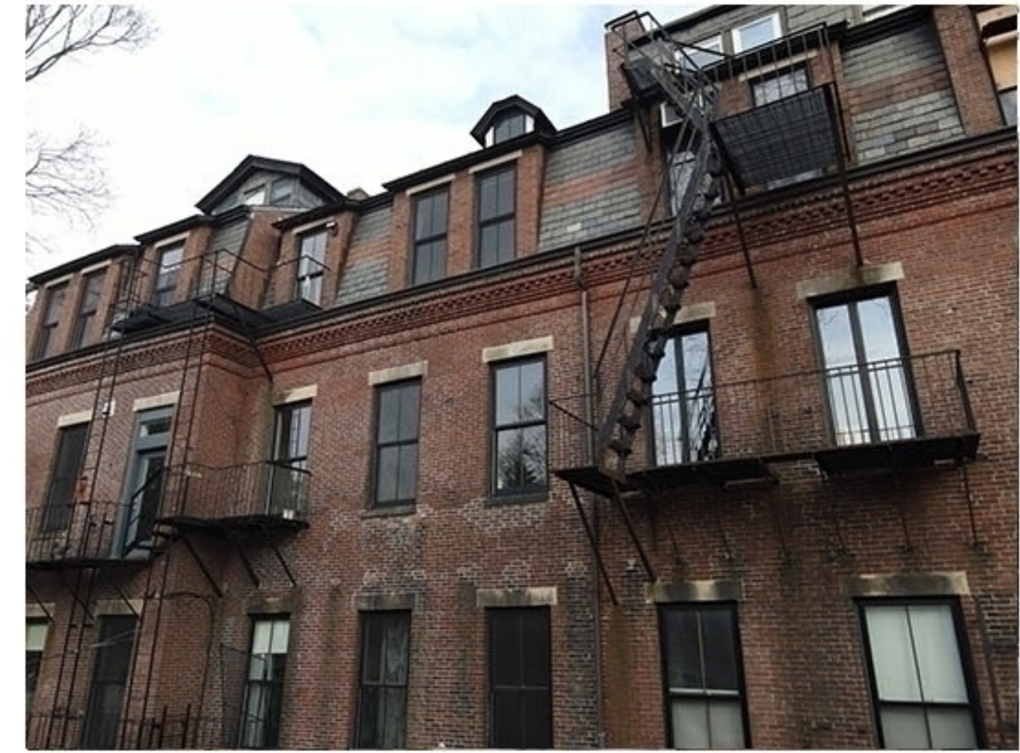
3 - REAR YARD VIEW UP, EXISTING
