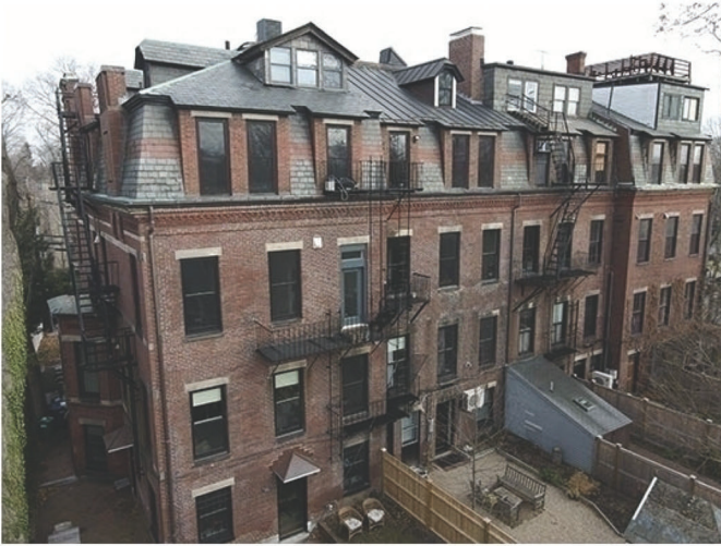
1 - NORTHWEST CORNER, EXISTING
