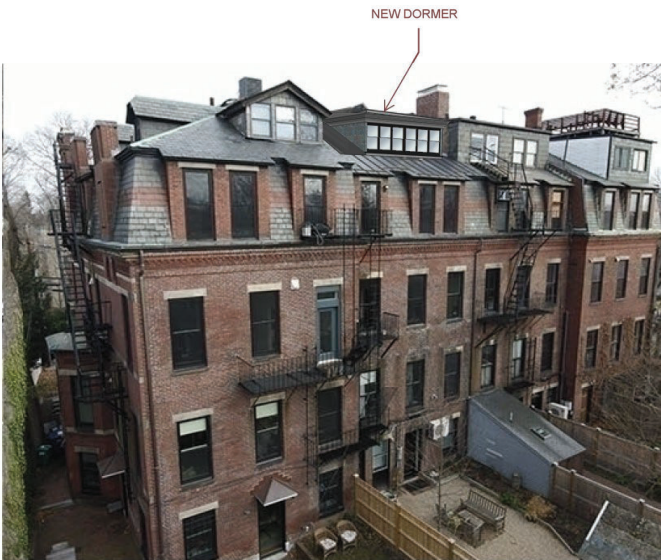
4 - NORTHWEST CORNER WITH DORMER / TERRACE
