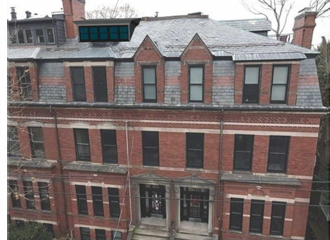
6 - VIEW UP TO ROOF WITH DORMER
