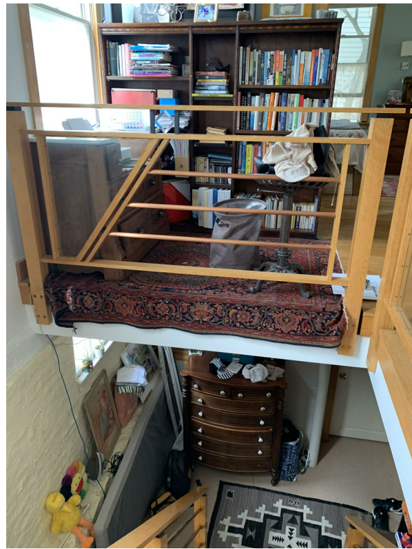
IMG 1: REMOVE EXISTING GUARDRAIL AND REINSTALL AT CATWALK
