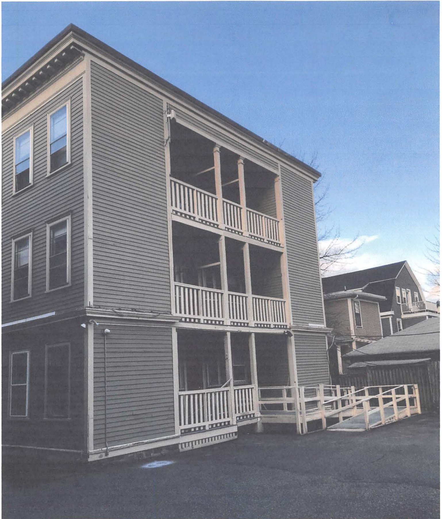
6 Sacramento St Handicap Ramp - located in the parking area
