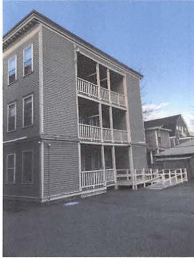
Handicap Ramp - located in the parking area
