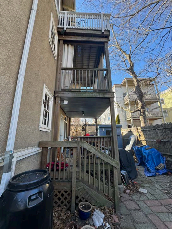
73 Fayette Street - views of the rear porch
