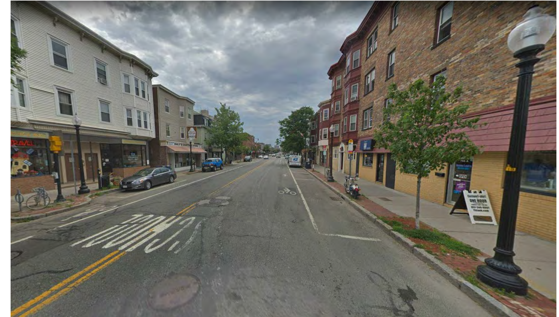
VIEW TOWARDS SITE FROM BERKSHIRE ST @ CAMBRIDGE ST
