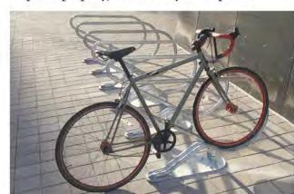
Acceptable racks, like the Inverted U," "Swerve," and "Post and Ring" racks, have two-point support and fit a variety of cicycle types. Custom lesigns and "artistic" acks can also be used, provided they meet the performance criteria for bicycle racks.
