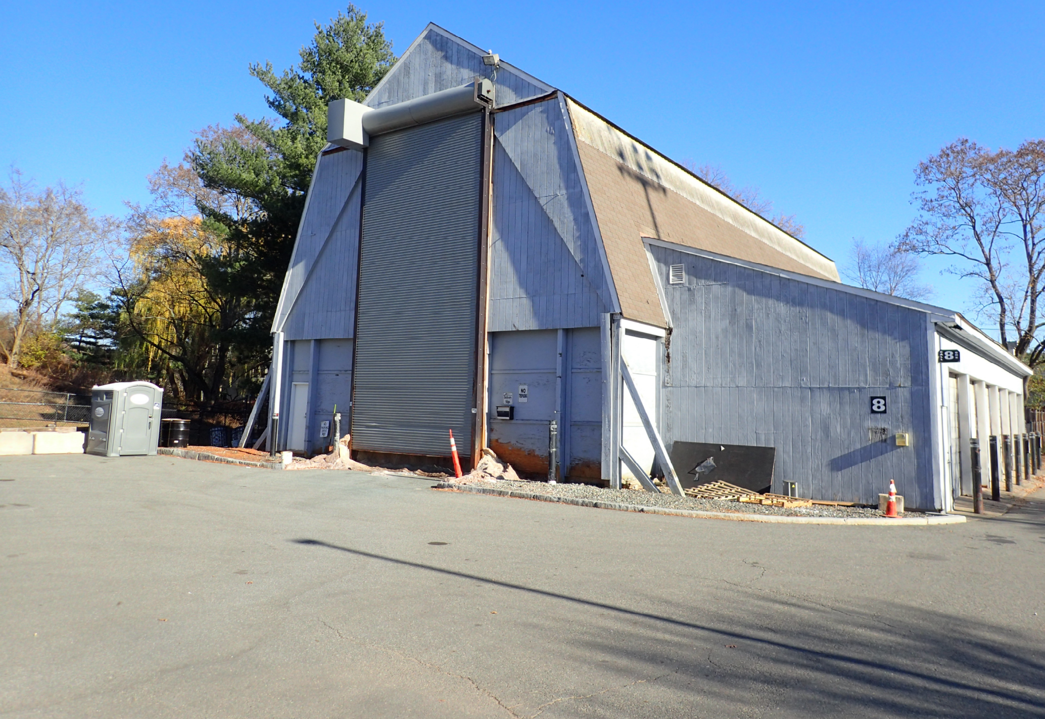
PHOTO 1 FRONT OF EXISTING SALT SHED
