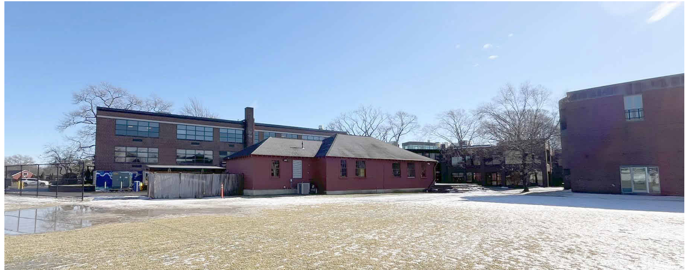
Existing Woodshop Building view of west facade from field
