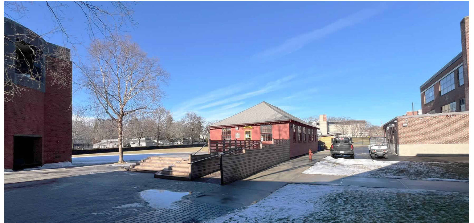
Existing Woodshop Building view from academic courtyard
