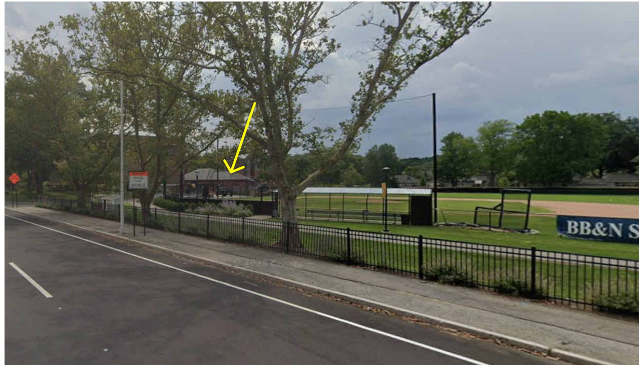
Existing Woodshop Building view from street
