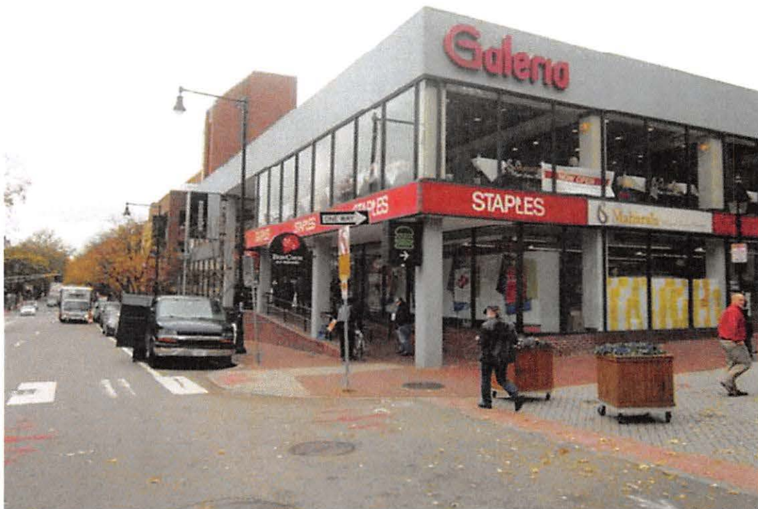
Fig 2 – View of N.E. corner of building
