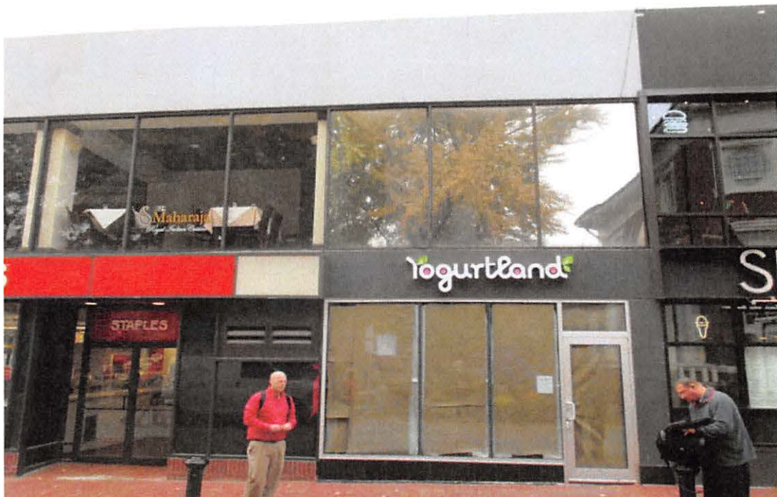
Fig 6 – Storefront adjacent to staples.
