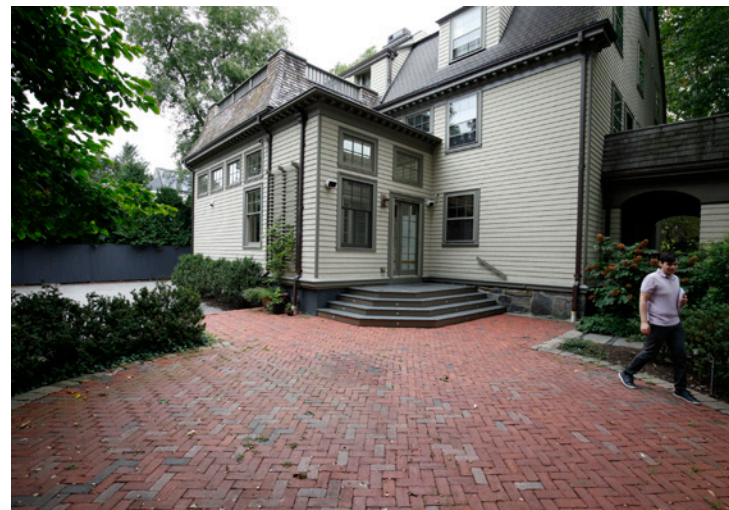
VIEW FROM PATIO LOOKING NORTHEAST (2022 - PRE-CONSTRUCTION)
