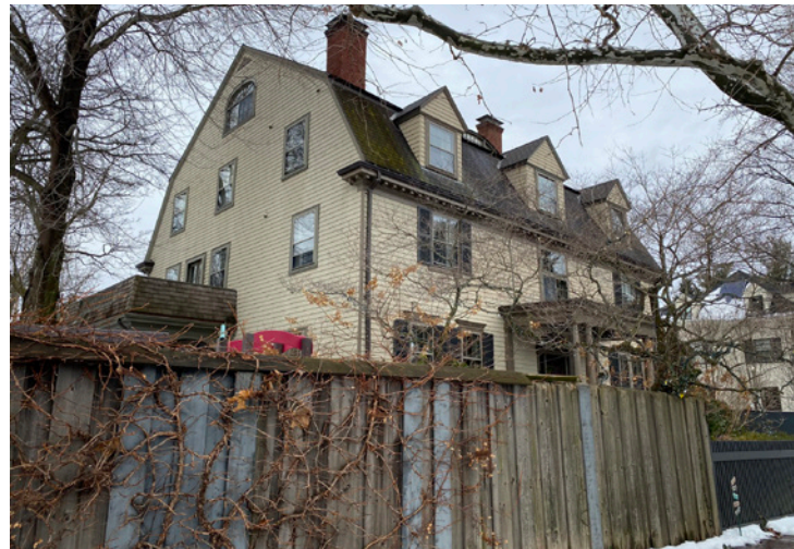
VIEW FROM SIDEWALK ON IRVING STREET LOOKING NORTHWEST (2022 - PRE-CONSTRUCTION)
