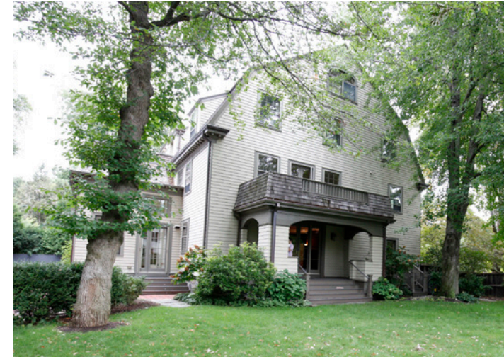
VIEW FROM SIDE YARD LOOKING NORTHEAST (2022 - PRE-CONSTRUCTION)
