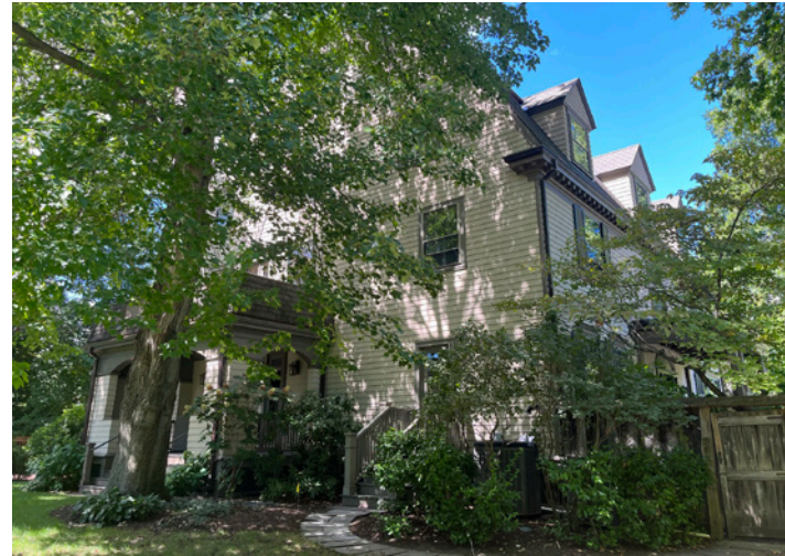
VIEW FROM SIDE YARD LOOKING NORTHWEST (2022 - PRE-CONSTRUCTION)
