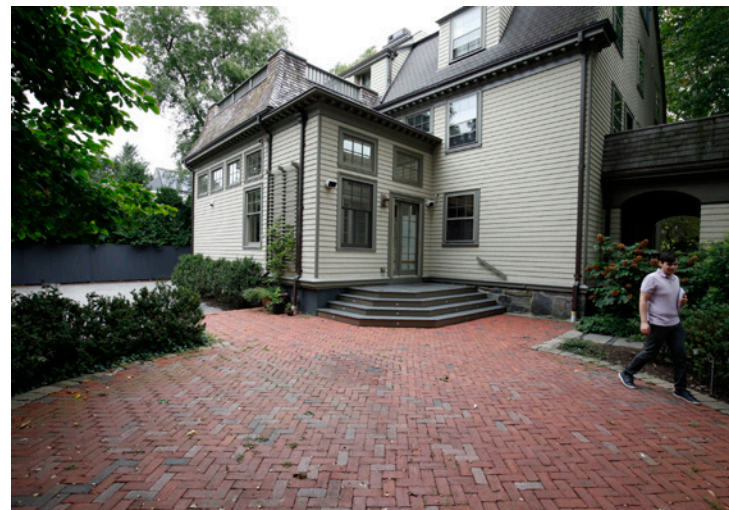
VIEW FROM PATIO LOOKING NORTHEAST (2022 - PRE-CONSTRUCTION)
