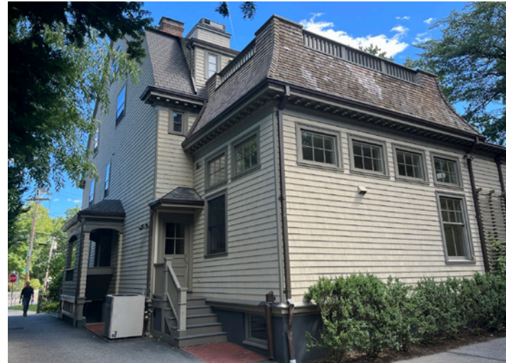
VIEW FROM THE DRIVEWAY LOOKING NORTHEAST (2022 - PRE-CONSTRUCTION)
