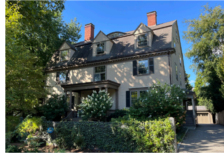
VIEW FROM SIDEWALK LOOKING WEST (2022 - PRE-CONSTRUCTION)
