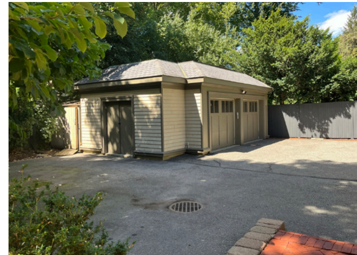
VIEW OF GARAGE LOOKING NORTHWEST (2022 - PRE-CONSTRUCTION)
