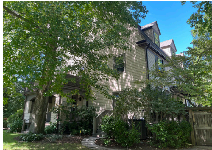
VIEW FROM SIDE YARD LOOKING NORTHWEST (2022 - PRE-CONSTRUCTION)
