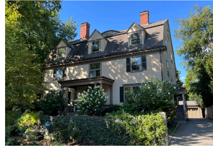
VIEW FROM SIDEWALK LOOKING WEST (2022 - PRE-CONSTRUCTION)
