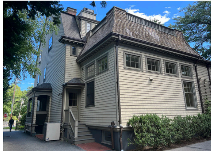
VIEW FROM THE DRIVEWAY LOOKING NORTHEAST (2022 - PRE-CONSTRUCTION)
