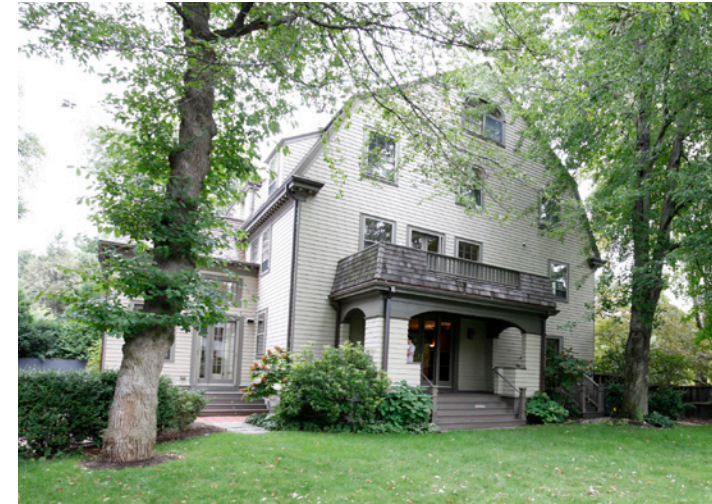
VIEW FROM SIDE YARD LOOKING NORTHEAST (2022 - PRE-CONSTRUCTION)
