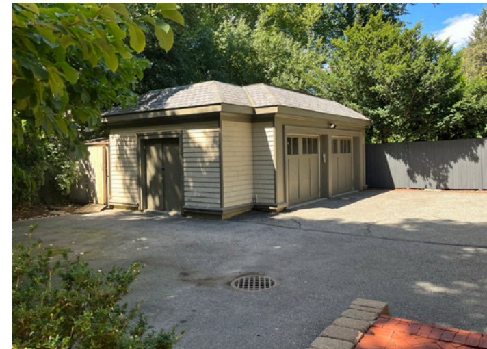
VIEW OF GARAGE LOOKING NORTHWEST (2022 - PRE-CONSTRUCTION)
