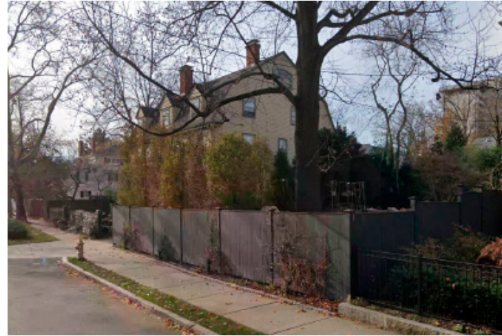
VIEW FROM SIDEWALK ON IRVING STREET LOOKING SOUTH (2022 - PRE-CONSTRUCTION)
