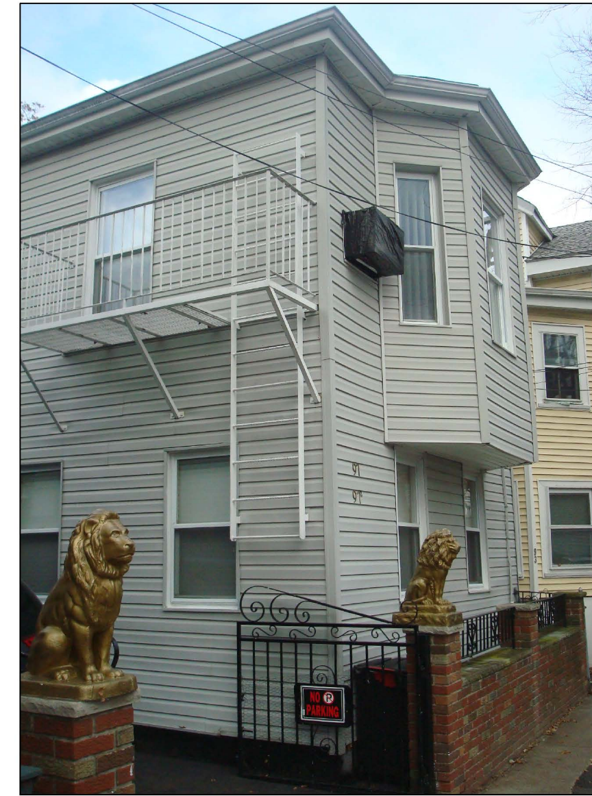
6 EXISTING SIDE VIEW 1/4" = 1'-0"
