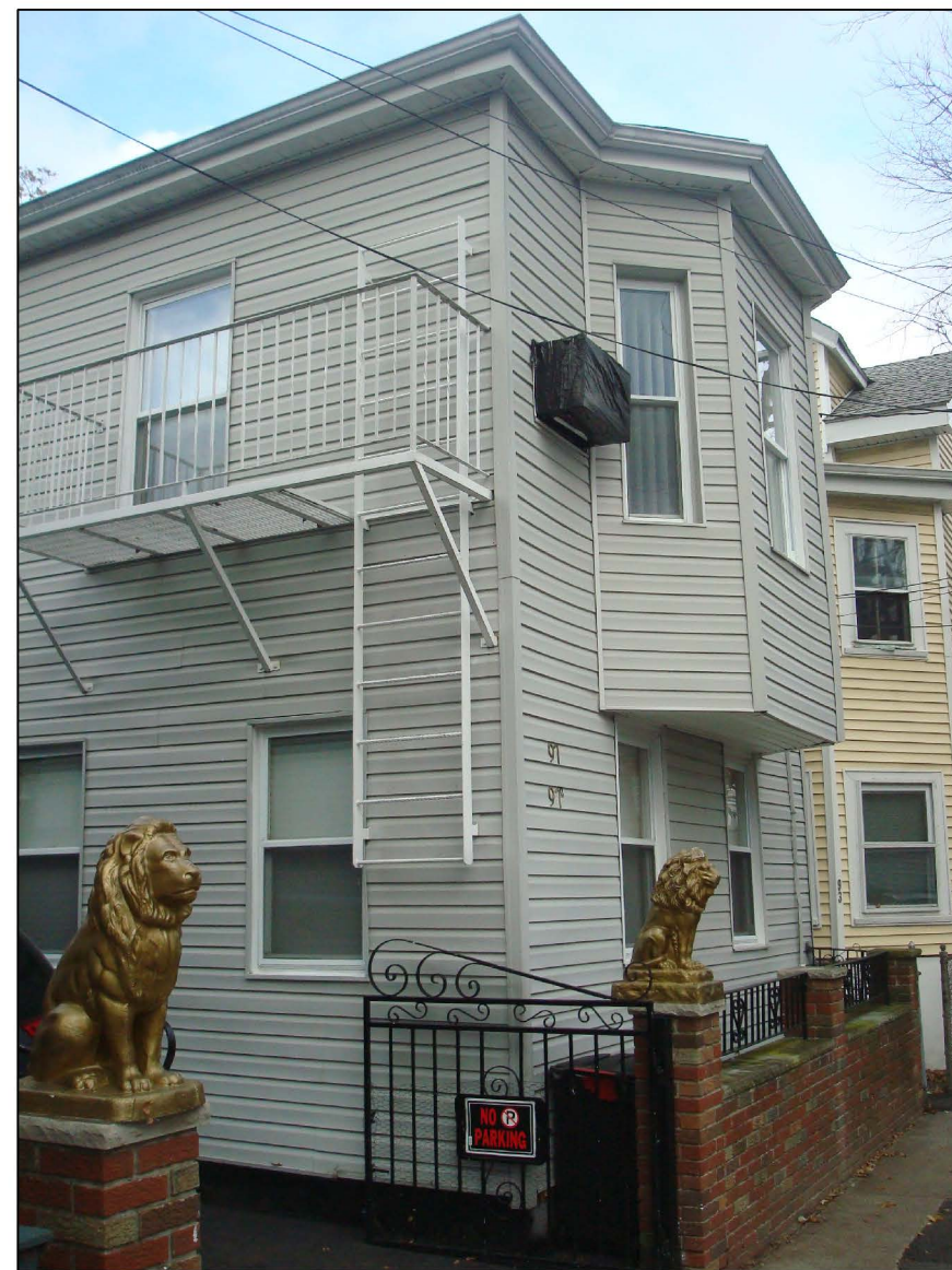
6 EXISTING SIDE VIEW 1/4" = 1'-0"
