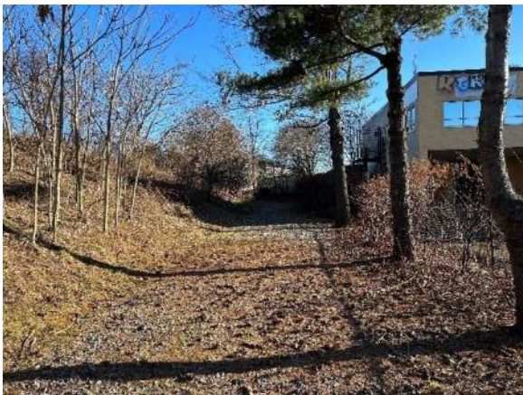
Photograph #15 Southeastern facing slope along vent trench showing woody growth on slope.
