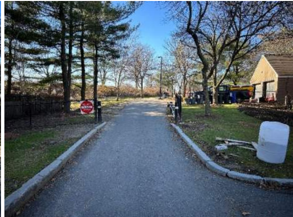
Photograph #2 Sherman Street Entrance to Danehy Park – Looking west.
