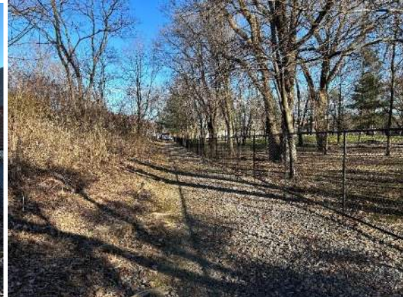
Photograph #20 Vent trench with Southeastern slope. Slope is overgrown with trees and woody growth. A desire path is shown along the base of the slope.
