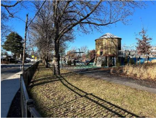
Photograph #41 Universal Design Playground at southern corner of site at the corner of Field Street and Garden Street.
