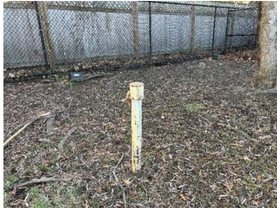
Photograph #40 MMW-4 landfill gas monitoring well is in very good condition.
