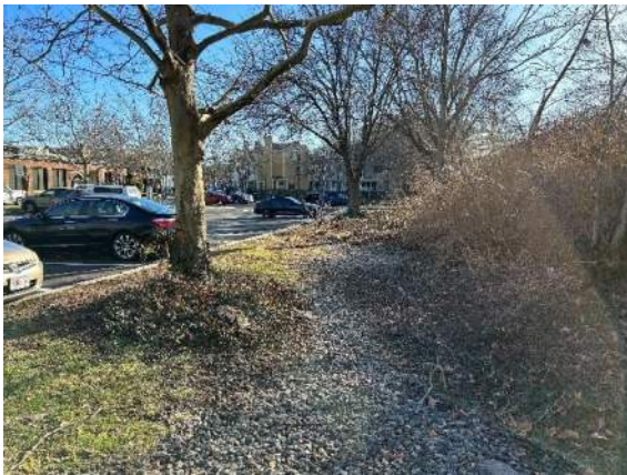
Photograph #23 Vent trench disguised as a dry stream bed on eastern side along Sherman Street Parking lot. Ground cover vegetation has spread into vent trench.
