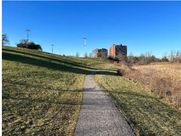
Photograph #28 Northeast slope with pond looking north.
