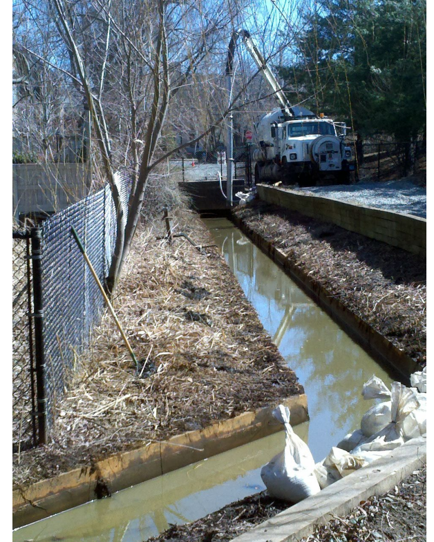
Photo from flood alleviation work
