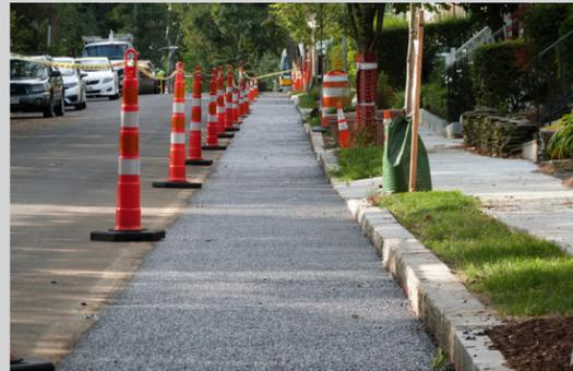
Porous pavement installation.
