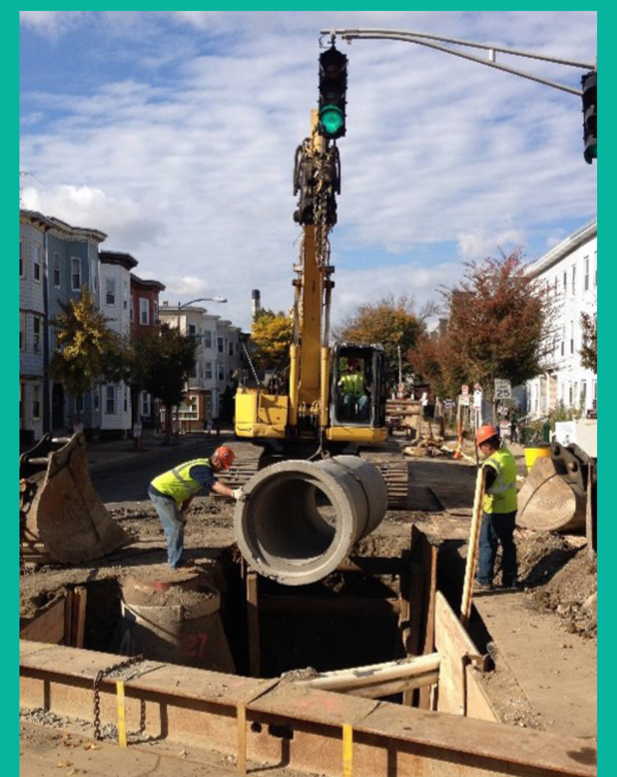
Installation of pipe
