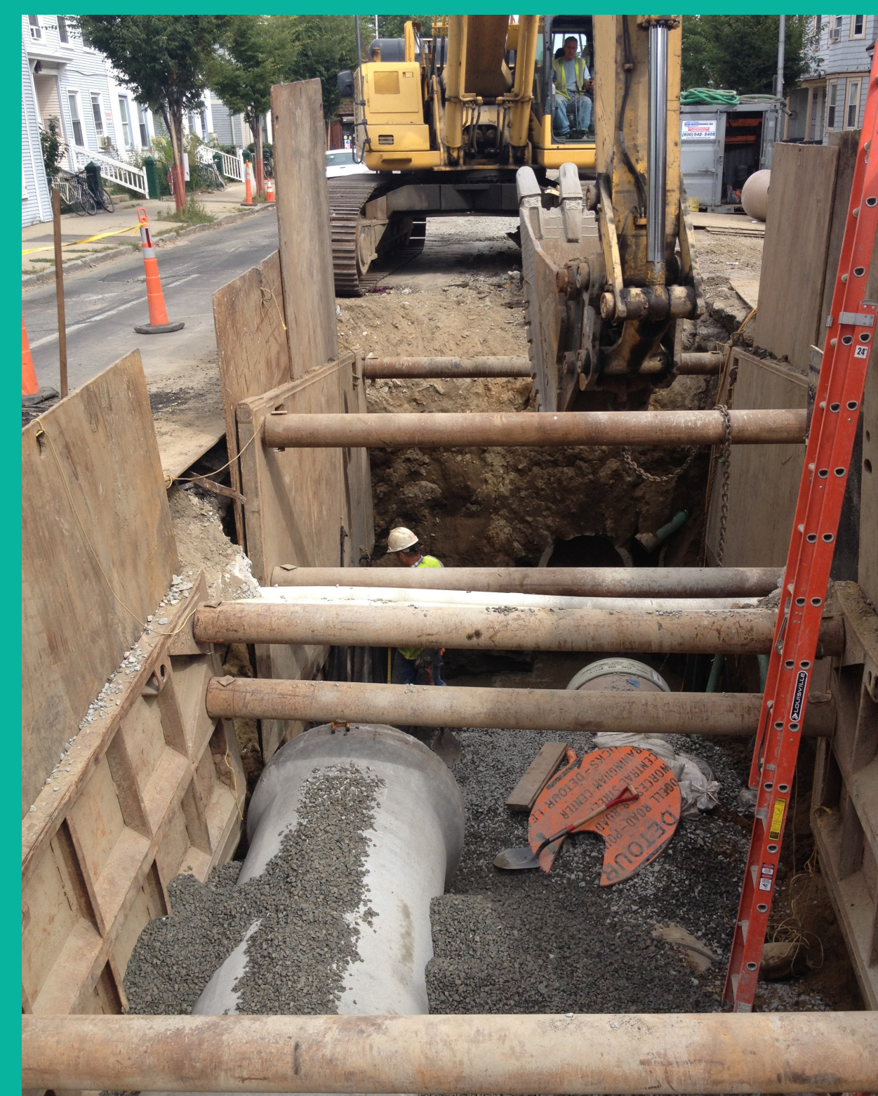
Trench with shoring
