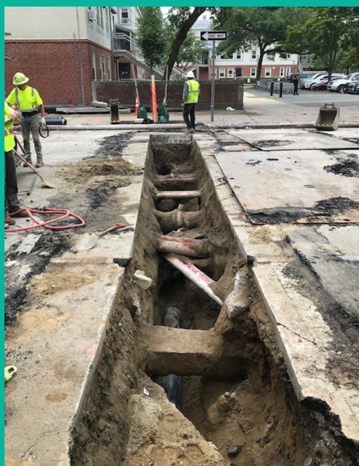
Existing subsurface utilities
