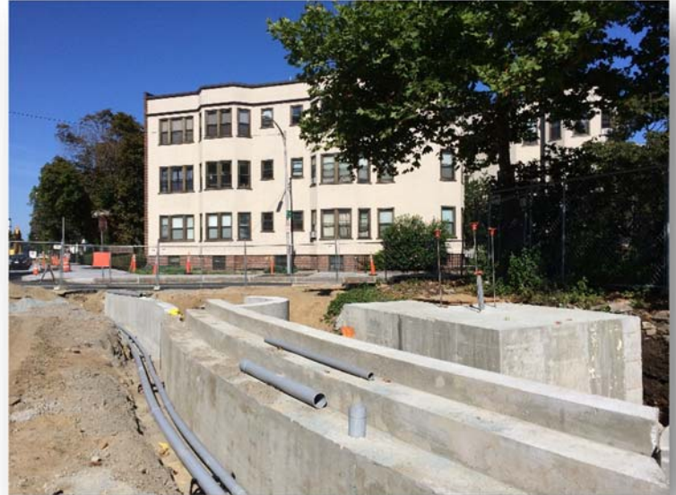
Installation of stairs at Cronin Park
