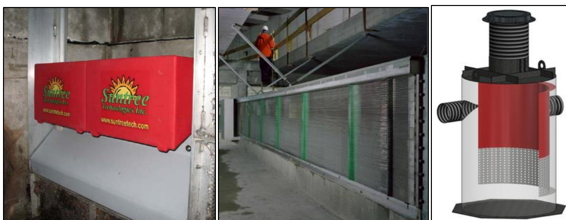
Figure 5: Dynamic Baffle (L), Mechanically Cleaned Screen (C), and Hydrodynamic Separator (R)
