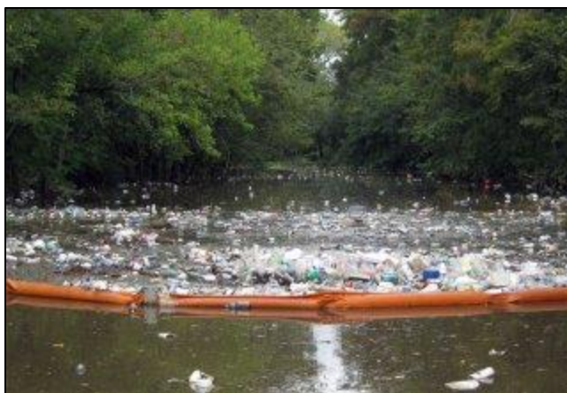
Figure 7: Containment boom floating on water surface. Floatables are trapped on one side of the boom.
