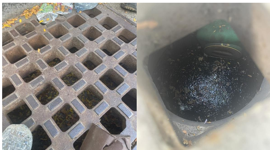
Figure 18: (L) Catch Basin D45CBN2013 was found to be full of debris with floatable options scattered across the grating. (R) Catch basin D45CBN2019 was the only CB inspected that was connected to storm water pipes upstream of the CAM401A outfall with a hood installed.
