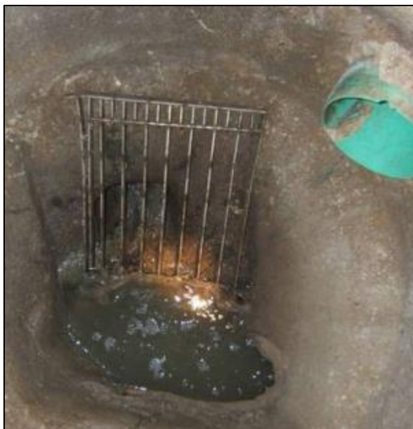
Figure 4: Example bar screen installation within a combined sewer system manhole
