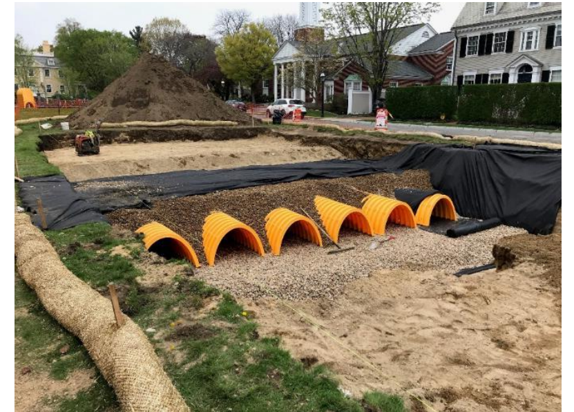
Longfellow Park – Underground infiltration
