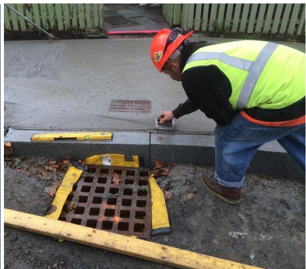
Silt sack installed in a catch basin to manage stormwater pollution during construction
