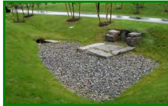
Infiltration swales
