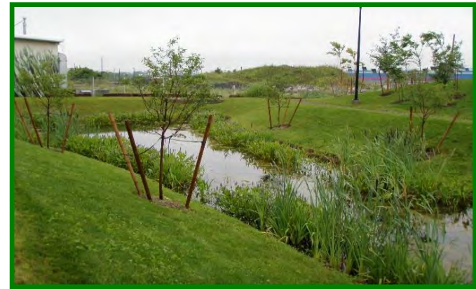
Infiltration swales
