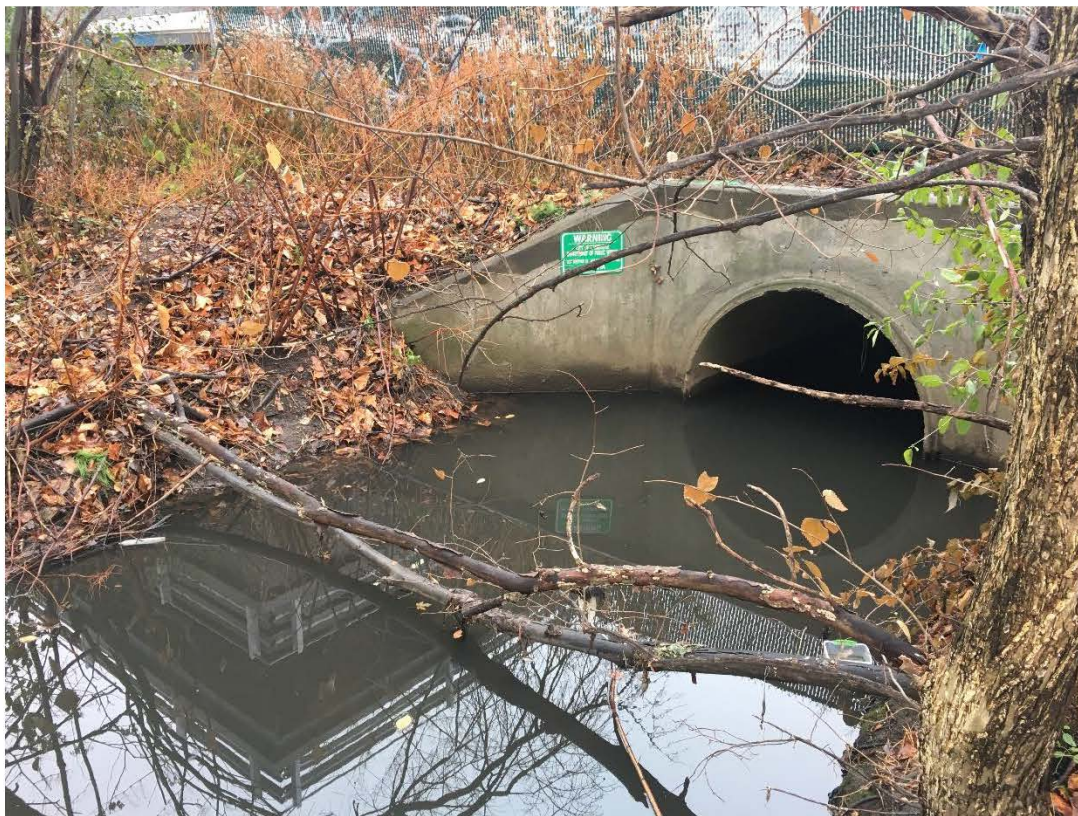
Photo 2: View facing south of CAM401A outfall.
