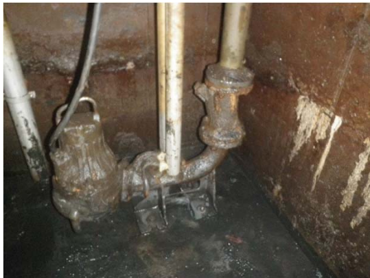
P2 Pump chamber after removal of sediments
