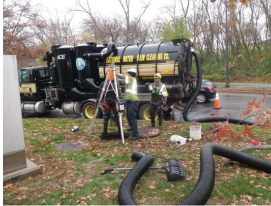
P1 Cleaning crew preparing to enter pump chamber
