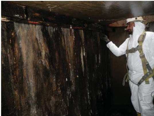
P7A Looking downstream at wooden bulkhead leading to 4'x12' culvert
