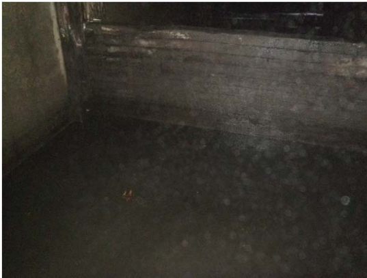
P7A Looking upstream before removal of 3' high wooden CSO weir
