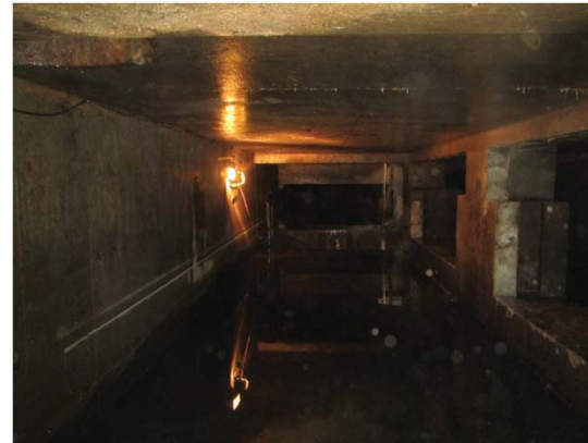
P4B Looking upstream after removal of 3' high wooden CSO weir
