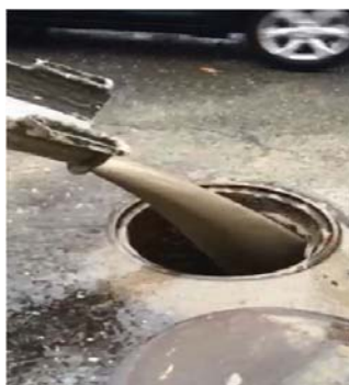
P10 – Flow-filling into manhole On MWRA's 48" sewer
