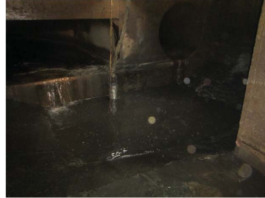
P6B Sumps restored after removal of wooden CSO weir
