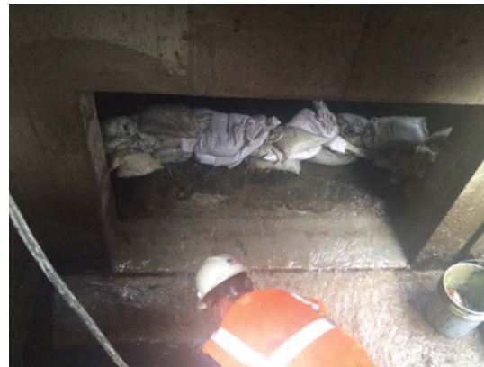
P14 Bulkhead removed between 72" drain and 4'x8' box culvert
