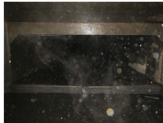
P7B Looking downstream at 4'x12' culvert after removal of wooden bulkhead
