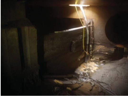
P6A Looking upstream at sumps before removal of wooden CSO weir
