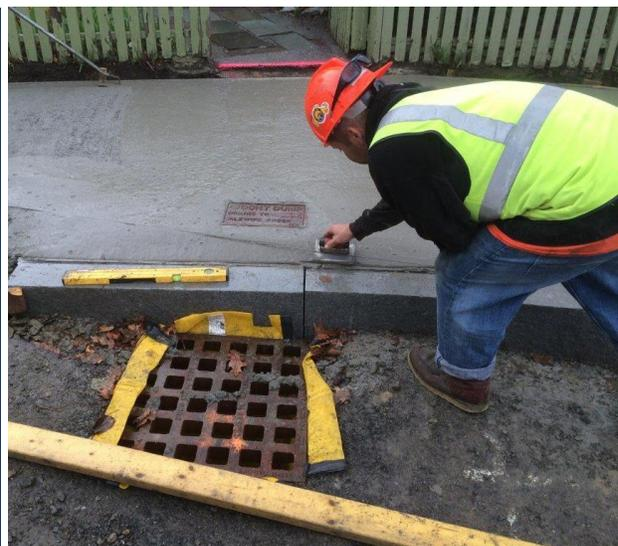
*Silt sack installed in a catch basin to manage stormwater pollution during construction*
