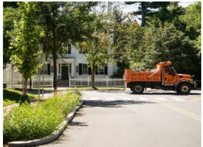
Installation of a rain garden to treat stormwater before it enters the drainage system as part of a sewer separation project.
