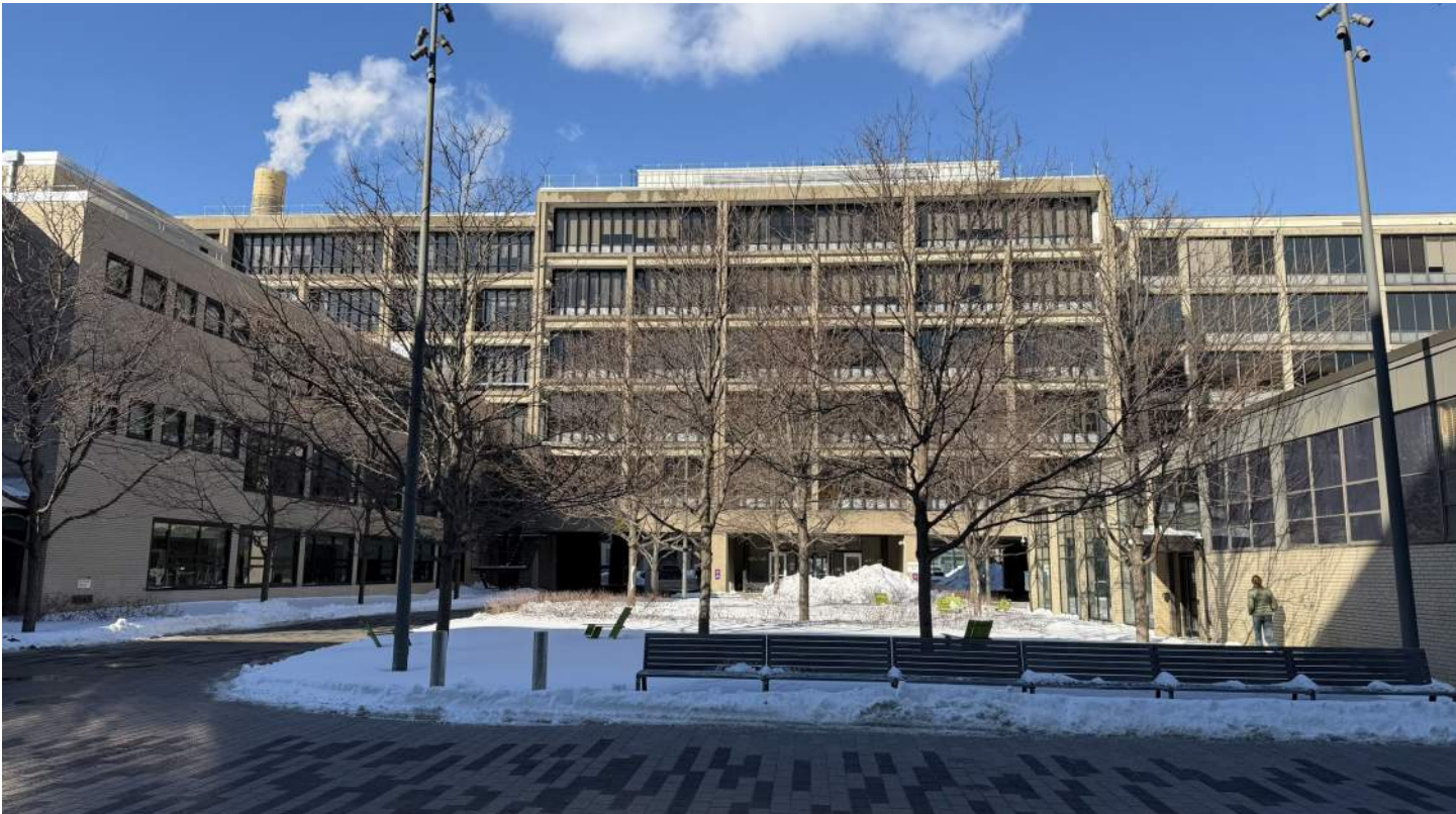
L. Rafael Reif Innovation Corridor View (South Facade)
