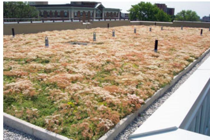
Figure 5. Green roof system [Source: [Toronto.ca](http://Toronto.ca) – Green Roofs - Green Roof at Ryerson University]
