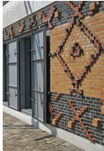
Figure 2a. Flood Protection Shutters [Source: City of Hamburg, Germany]
