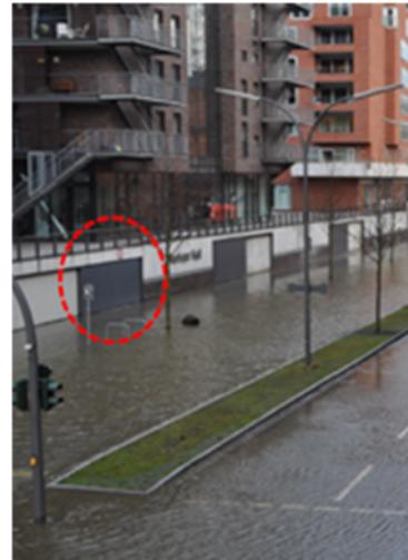
Figure 2b. Flood Protection Gates to achieve a Flood Protection Level [Source: HafenCity, Hamburg, Germany]
