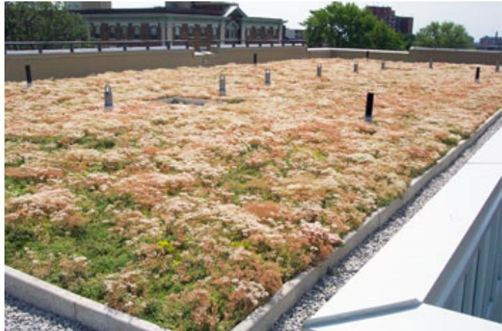
Figure 5. Green roof system [Source: Toronto.ca – Green Roofs - Green Roof at Ryerson University]
