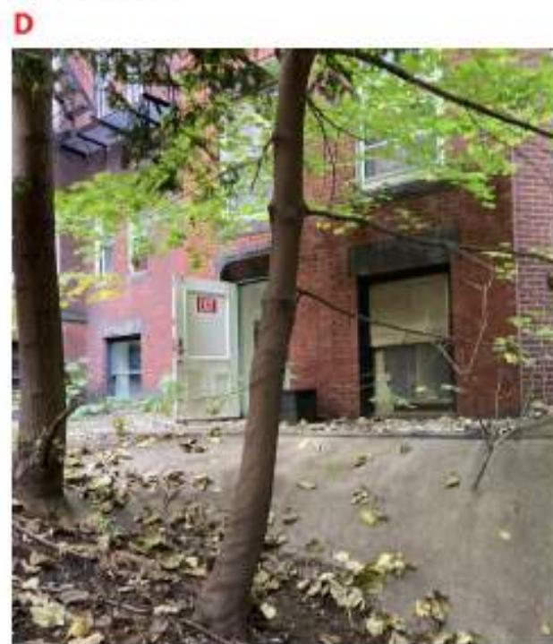
- EXISTING STEEP SLOPE NEEDS TO BE FLATTENED FOR ACCESSIBLE AND USABLE COURTYARD SPACE
