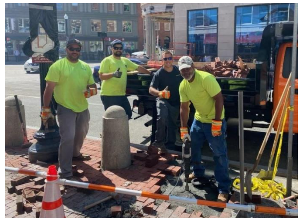
Brick repairs in Harvard Square
