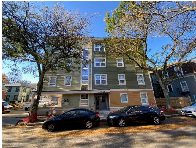
Squirrelwood, 88 units of newly constructed or rehabilitated units in The Port that will remain affordable in perpetuity
