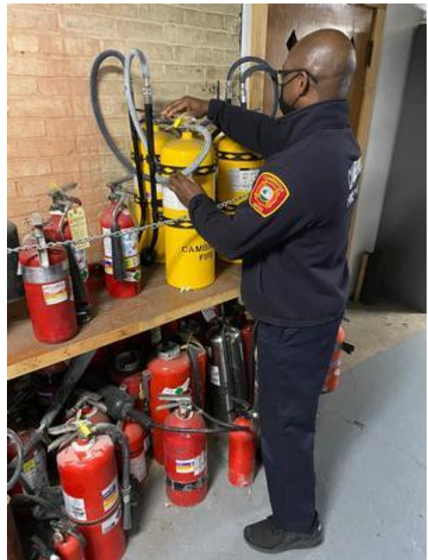
A member of Fire Prevention inspecting replacement fire extinguishers
