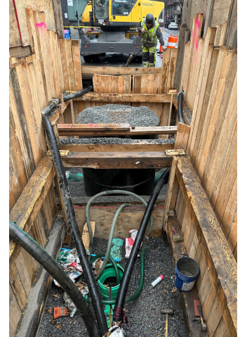
Replacement of a sewer manhole on Third Street
