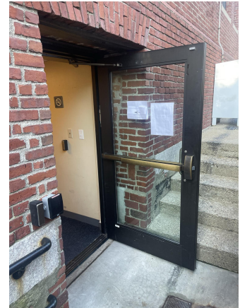
Physical security upgrade to secure employee entrance to city building
