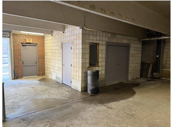
Concrete walls at First Street Garage
