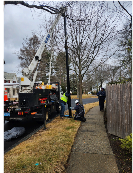
Workers installing a streetlight pole on Meadow Way
