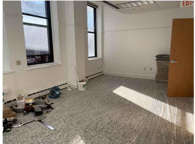
Building repairs work
