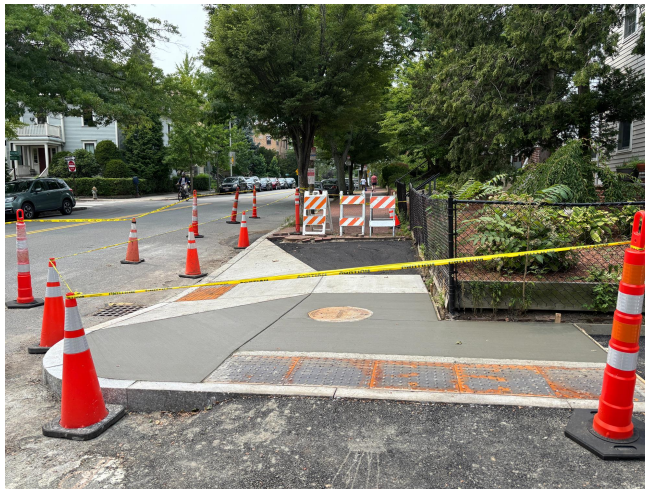
Sidewalk reconstruction on Maple Avenue
