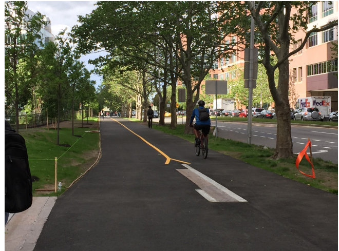
Completed portion of the Grand Junction Multi-Use Path along Galileo Galilei Way
