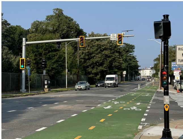
New two-way bike lane on Mt. Auburn Street at Aberdeen Avenue
