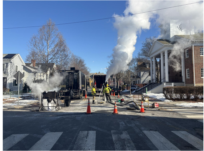
Sewer lining work at intersection of Beech and Orchard
