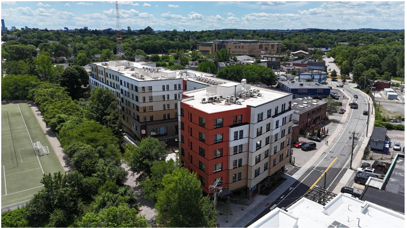
52 New Street completed
