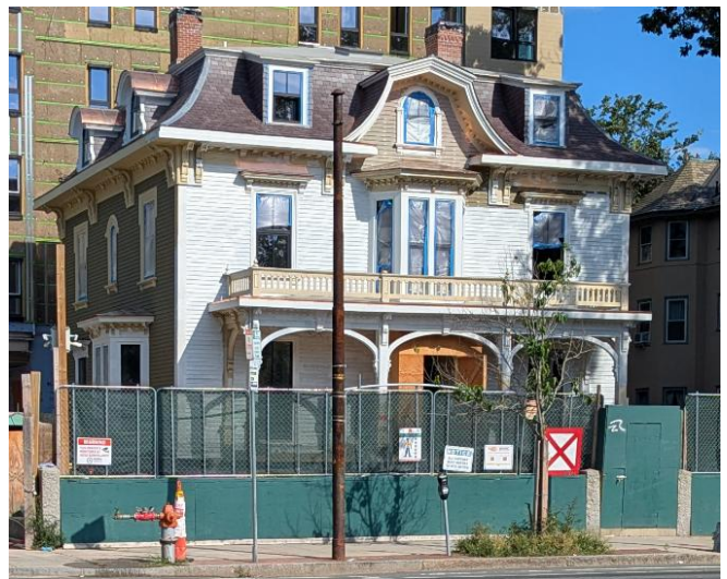
Restoration of 1627 Massachusetts Ave.
