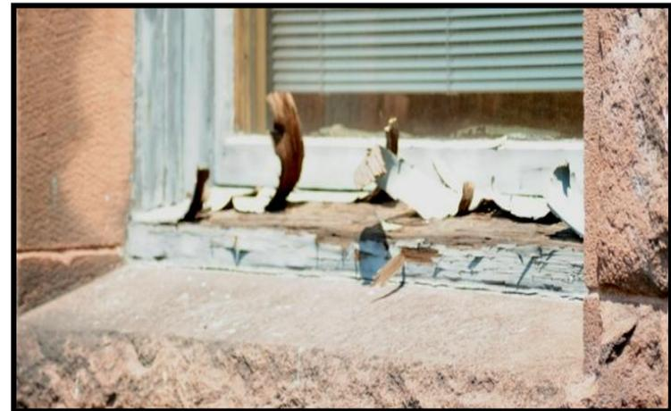
Window sills must be restored or replaced. Storm windows would minimize energy loss and allow retention of original sash.
