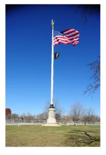
Flagstaff Park (1915). Funds would be used to restore the historic memorial flagpole in Flagstaff Park. The flagpole and base were originally installed in 1915 and have been damaged by the elements. The concrete base would be repaired, and the rotting wooden pole would be replaced to restore the flag and copper eagle finial to its original height. FY22 funding would supplement FY19 funding, which was expended for design and site preparation, including compression testing. (\$175,000)
