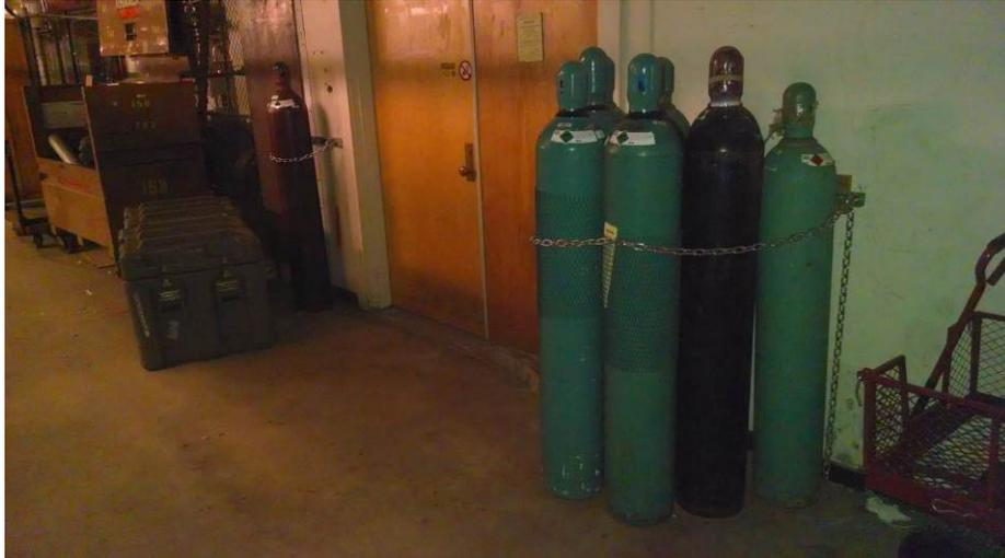
Lastly, what are the exposures? Although they are properly secured, these hydrogen and oxygen cylinders are directly in the vicinity of the electrical area and present exposure hazards in themselves.
