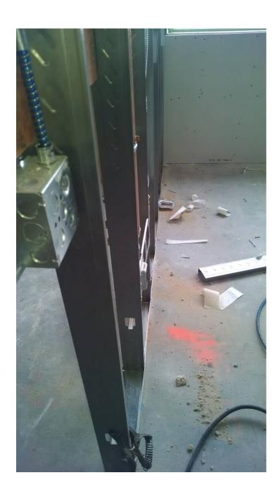
However the same wall viewed from the other side, you see that almost all of the stud bays have some type of obstruction, even electrical and plumbing for the adjoining room, even if its appears as a breachable wall! Out of the five stud bays shown, only one would allow sufficient room for a firefighter, fully geared to crawl through. The bottom line is <u>KEEP TRYING!</u>
