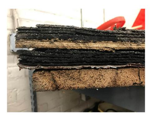
Truck companies are expected to get to the roof and vent but often run into obstacles such as this. Clearly a code violation. This photo is NOT from Cambridge, but could happen anywhere! Starting from the lowest layer – wood roof sheathing, metal roof, 3 layers of asphalt shingles, ½" plywood with another 3 layers of asphalt shingles.
