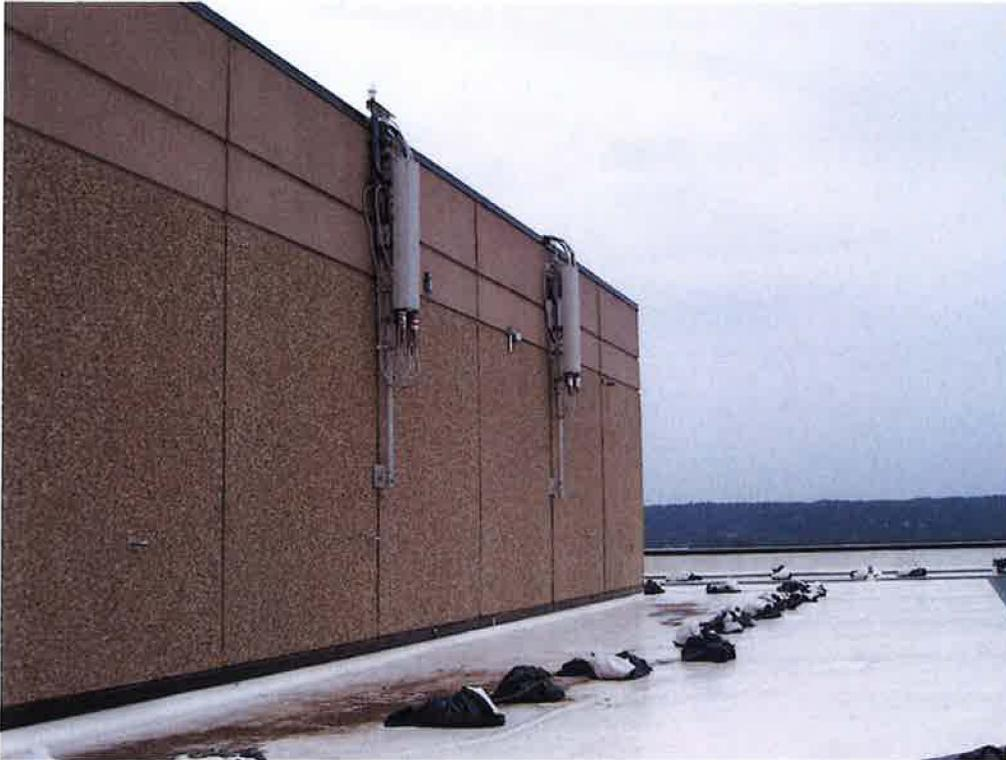
**Photo 1:** Sample photo illustrating the existing antennas secured to the building façade.
