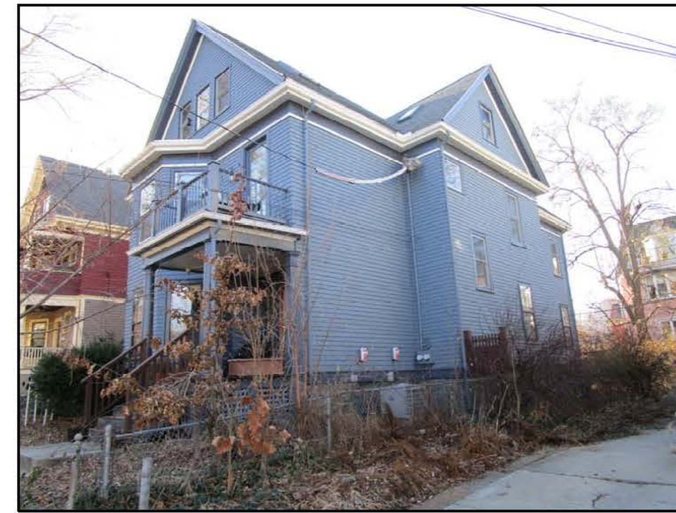
EXISTING FRONT RIGHT VIEW
