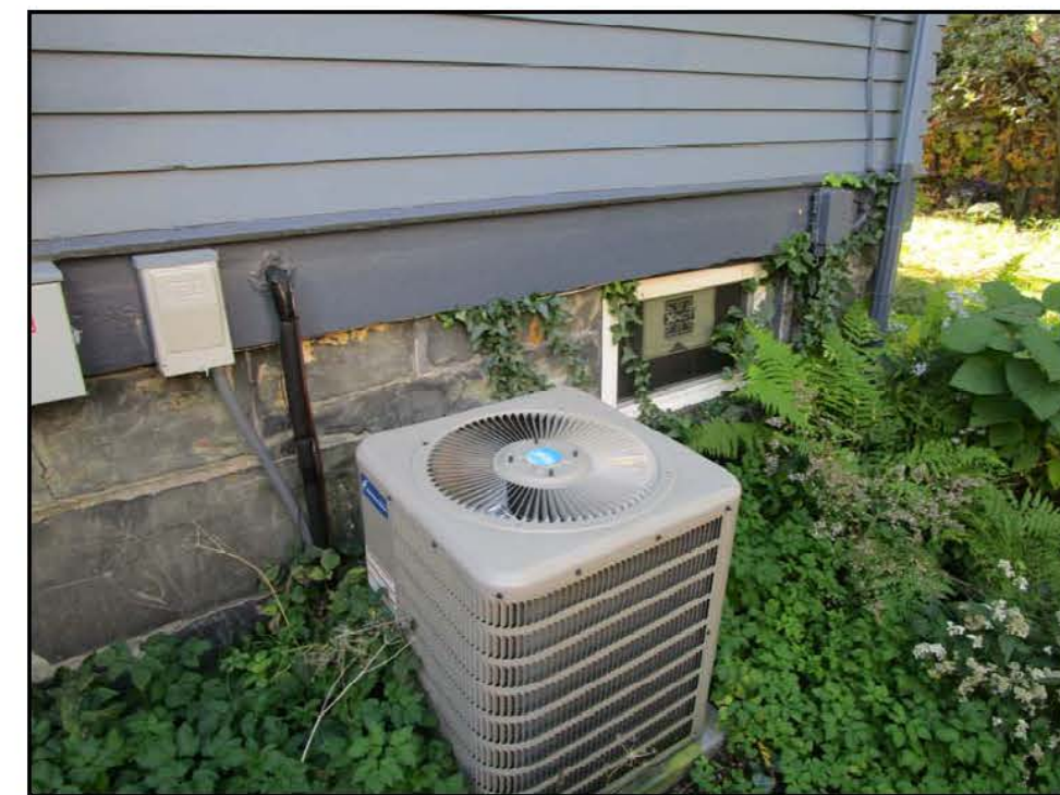
EXISTING NORTH ELEVATION (REAR WINDOW YARD SIDE)
