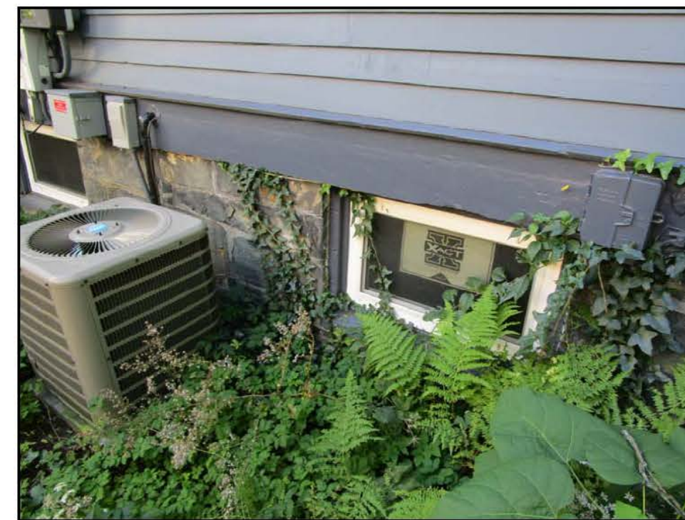
EXISTING NORTH ELEVATION (REAR WINDOW YARD SIDE)
